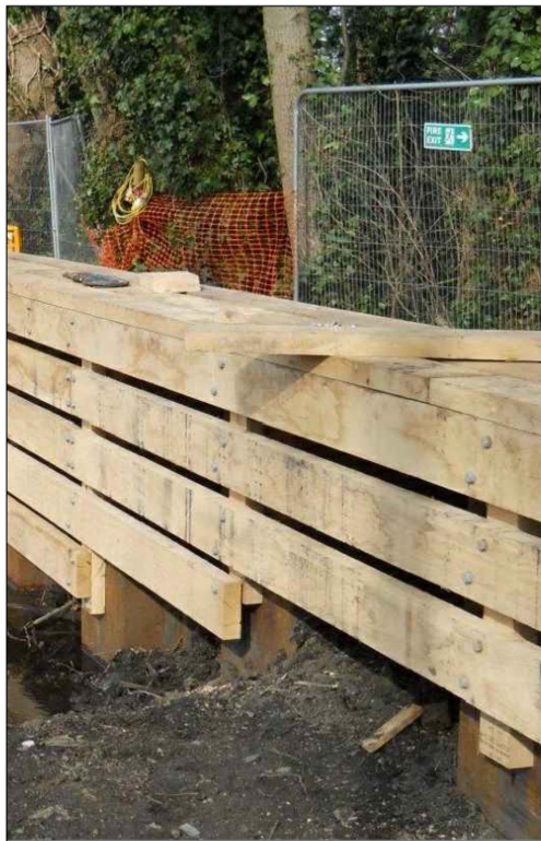
Timber Clad Sheet Pile Wall Not To Scale
