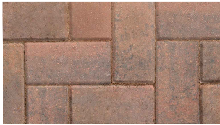
Paving Type: Standard concrete 'bridle' block paving
