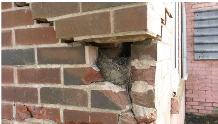
Figure 3-5: Damaged brickwork on the reception building
