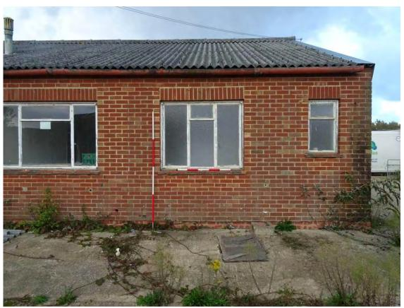
Plate 27. Detail of the southern elevation showing crinkle casements and brickwork
