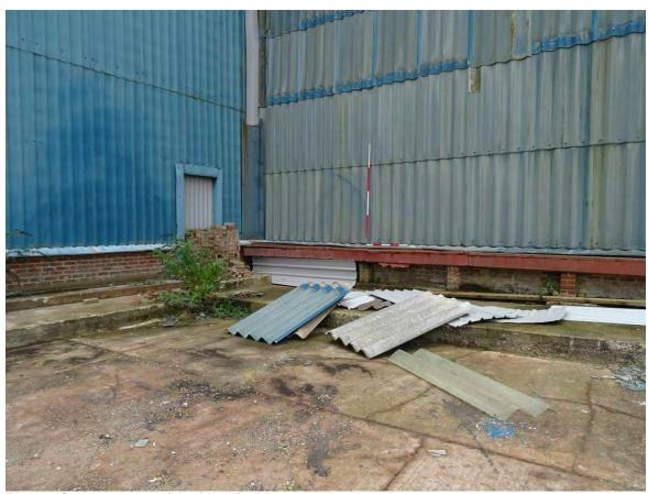
Plate 9. Corner section of the Main Building, showing the join between the two construction phases
