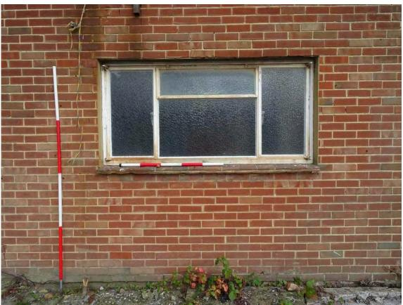
Plate 29. Detail of showing crinkle casement and surrounding brickwork
