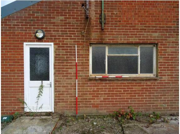
Plate 28. Detail of the western gable showing crinkle casements, UVPC door and brickwork
