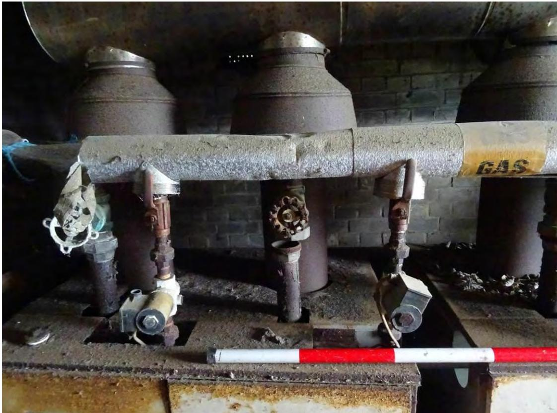
Plate 56. Valve system for the release of excess steam, located about the boiler system
