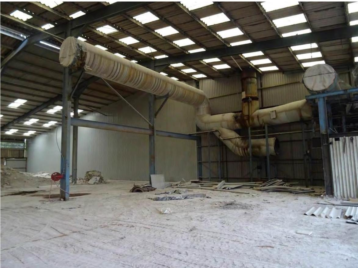
Plate 19. View showing redundant heating ducts and strut supports, looking NW
