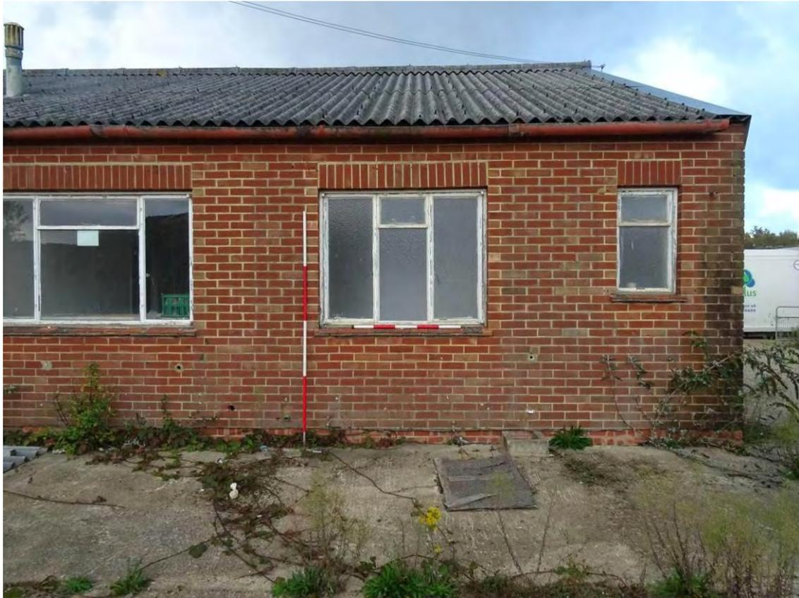
Plate 27. Detail of the southern elevation showing crinkle casements and brickwork
