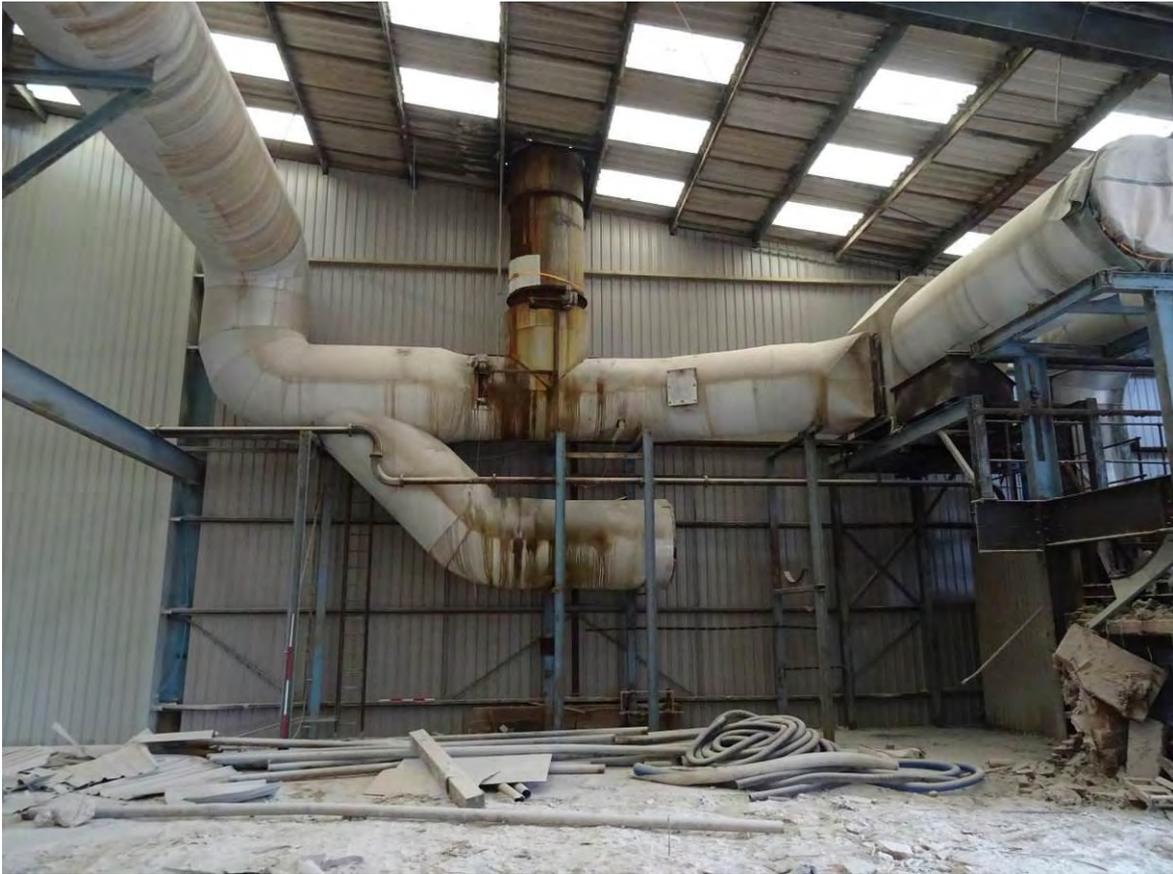
Plate 18. View showing redundant heating ducts and strut supports, looking north
