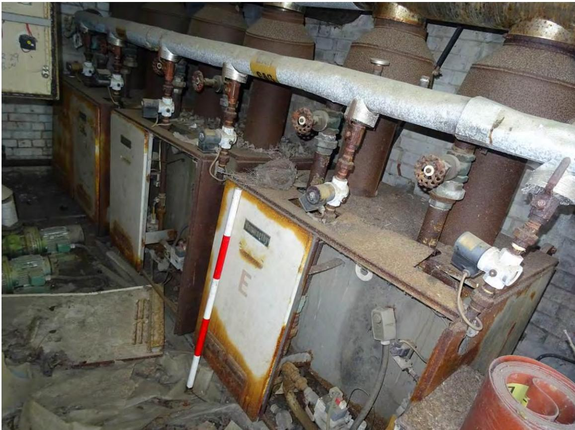
Plate 53. Internal view of the gas-fired boiler condensing range, looking SW
