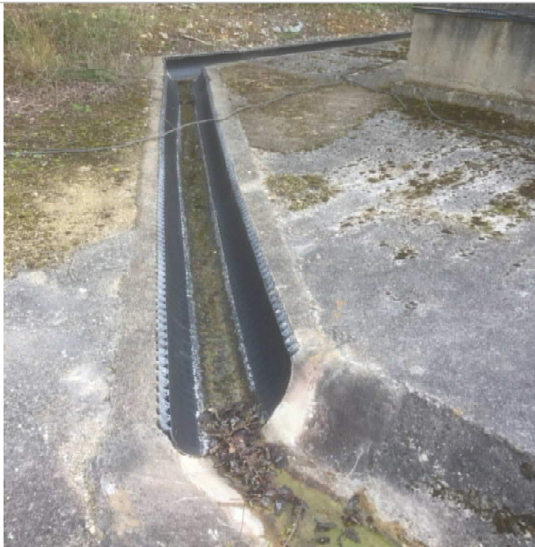
Photograph 2512/FRA/P4 - uncovered fuel interceptor
