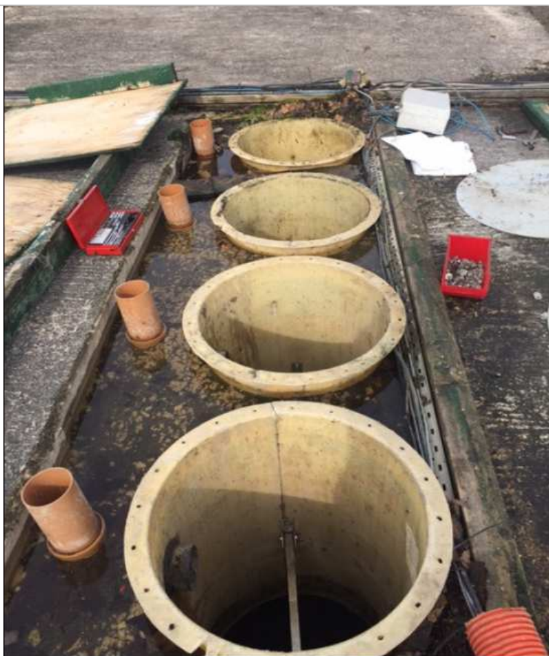
Photograph 2512/FRA/P4 - uncovered fuel interceptor
