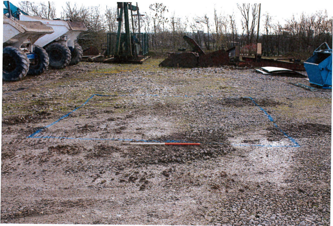
Fig. 3.1: Footprint of excavation area looking east
