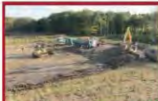
After the rig is dismantled, the primary stage of site remediation will be to take down the surrounding soil mounds and move the topsoil to the site centre.
