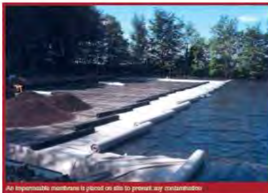
An impermeable membrane is placed on site to prevent any contamination
