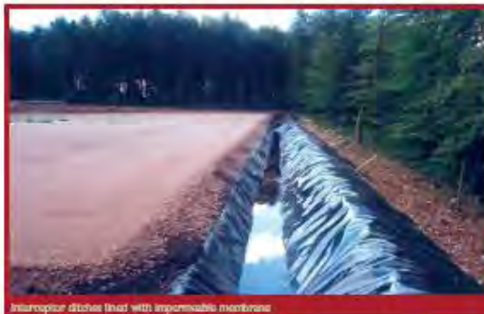
Interceptor ditches lined with impermeable membrane
