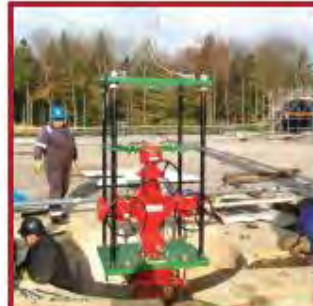
A 'Christmas tree' is installed at a well. This small unit consists of master and secondary valves to control and isolate the well.
