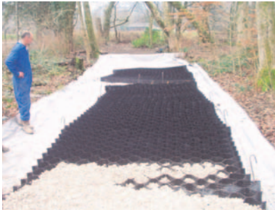
CellWeb during installation.
