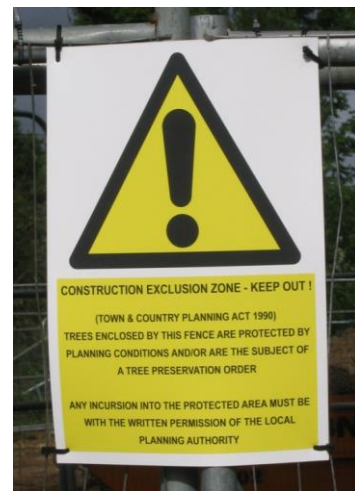
Figure 2 - Example of suitable warning sign affixed to protective barrier
