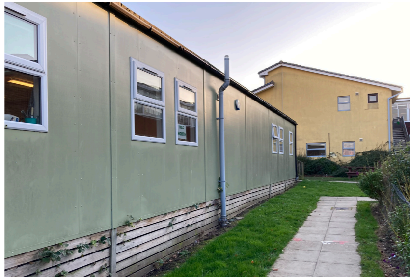
4. Existing surrounding school buildings
