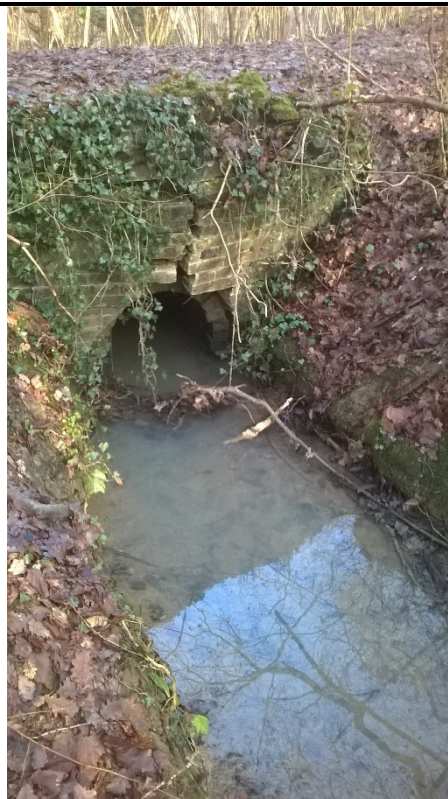
Photograph 4: Damaged culvert (western plot).
