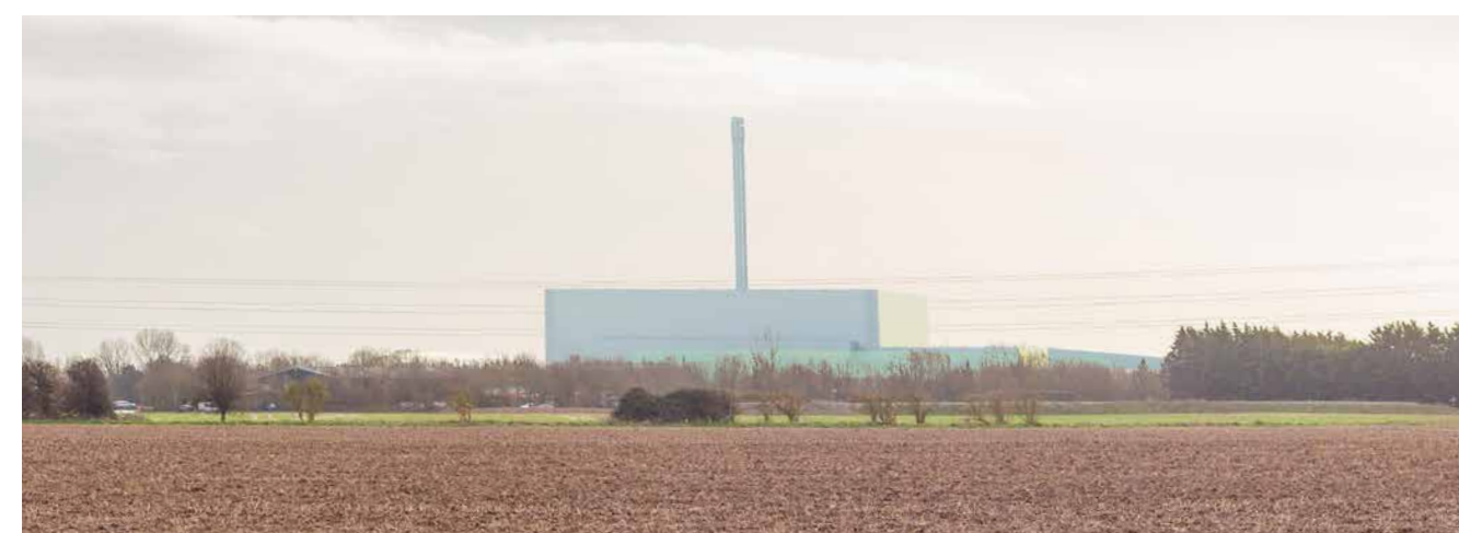
Figure 4.31 View from nearby PROW to the east of St Mary's Church, Yapton Radiused design
