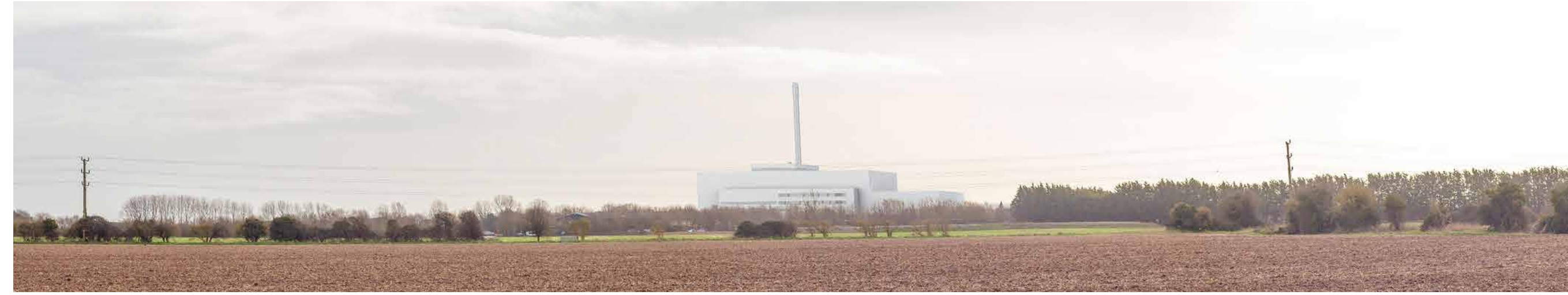
Figure 4.37 View from nearby PROW to the east of St Mary's Church, Yapton Proposed design
