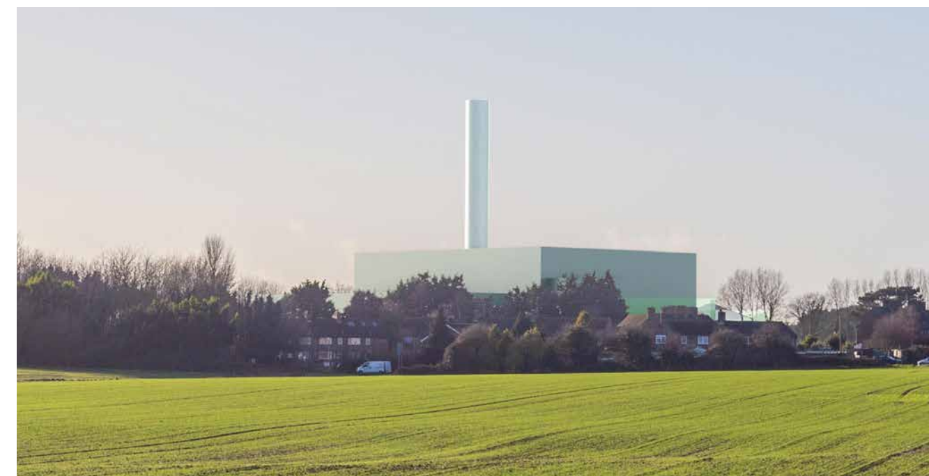
Figure 4.20 View from near St Andrew's Church Single 'cylindrical' stack
