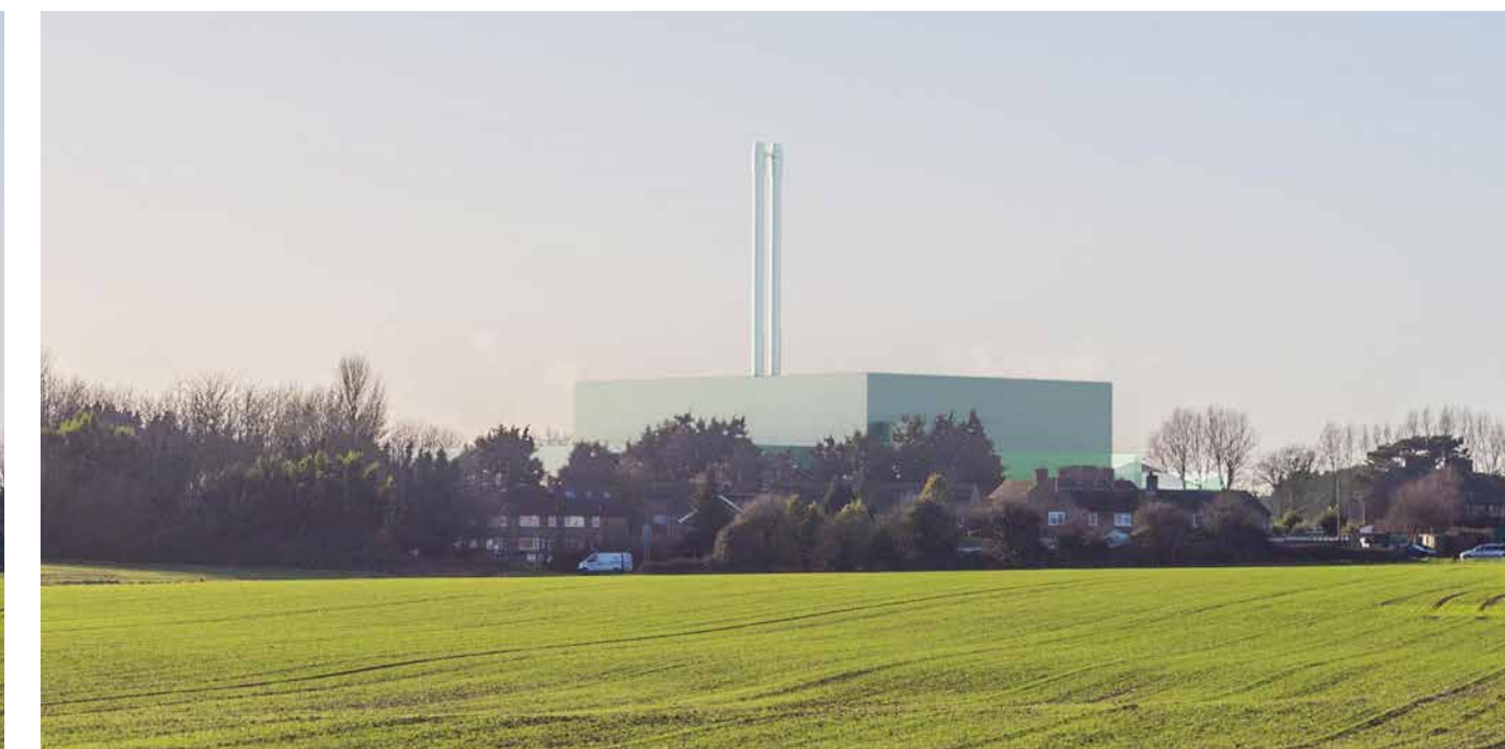
Figure 4.22 View from near St Andrew's Church Twin 'pencil' stacks
