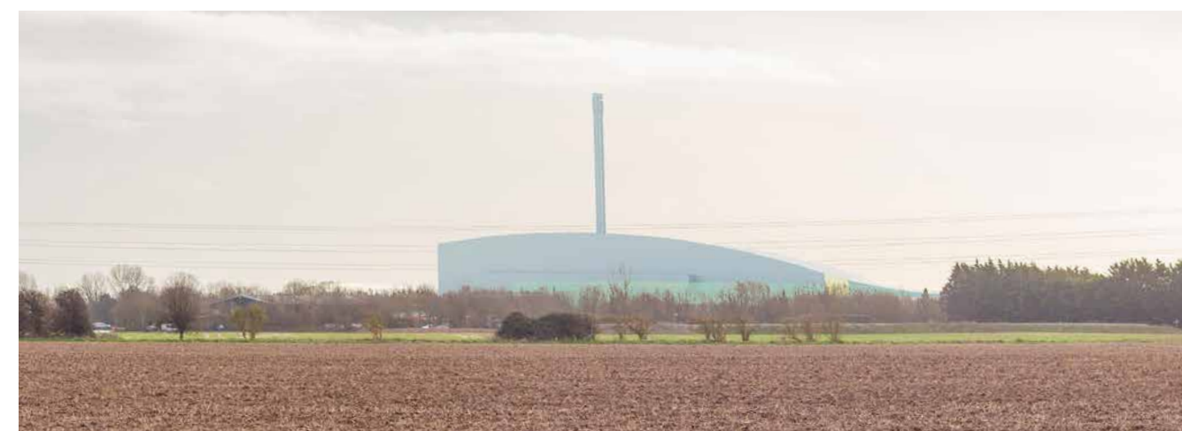
Figure 4.33 View from nearby PROW to the east of St Mary's Church, Yapton Curved design
