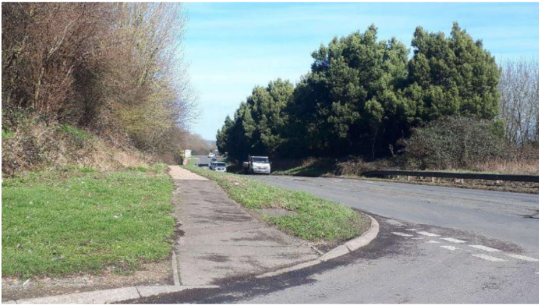
Photo C Ford Road showing existing VRS opposite site entrance
