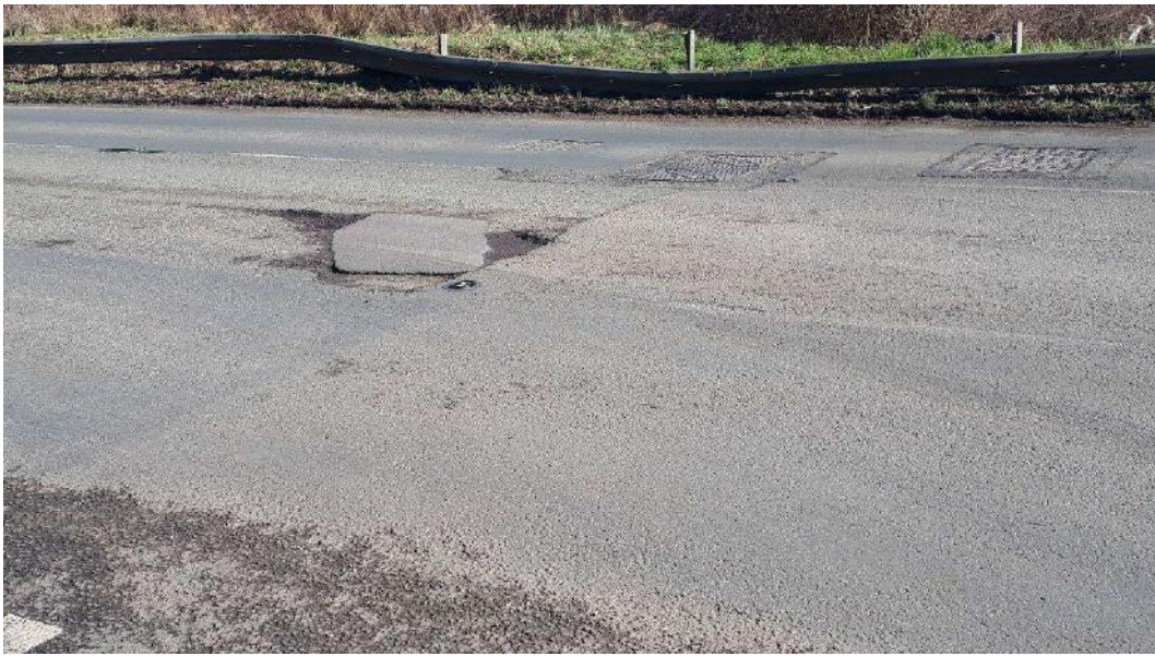
Photo K Ford Road carriageway markings illegible
