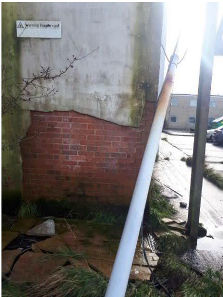
Photos A.7–A.9: Existing Drainage Features
