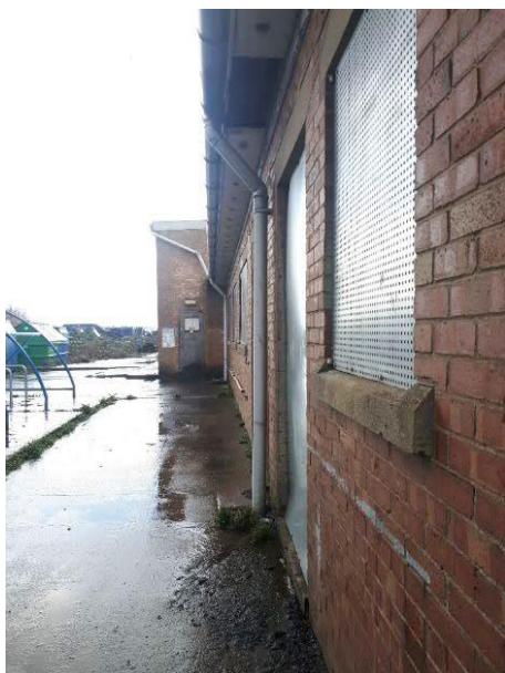
Photos A.3–A.6: Rainwater Pipes in Existing Buildings
