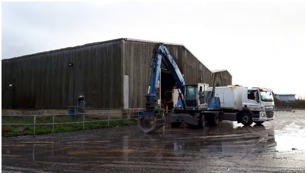
Photo 6. Main waste building
