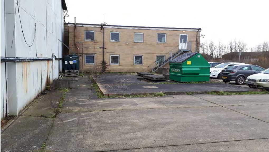
Photo 17. Former Location of 40,000 l Tank Containing Heating Oil (now Occupied by Green Bin)
