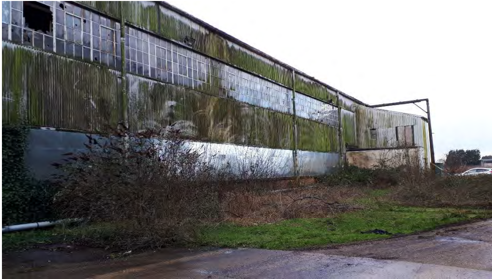
Photo 3. Hangar 1, facing southwards
