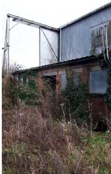
Photo 5. Smaller single storey bricked building on the northern side of Hangar 2
