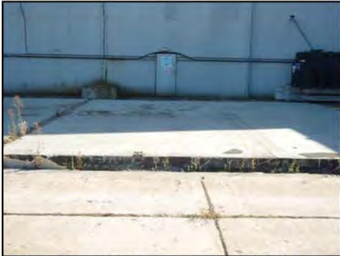
Plate 11: Location of former boiler house and associated gas oil tank (40,000 litres).
