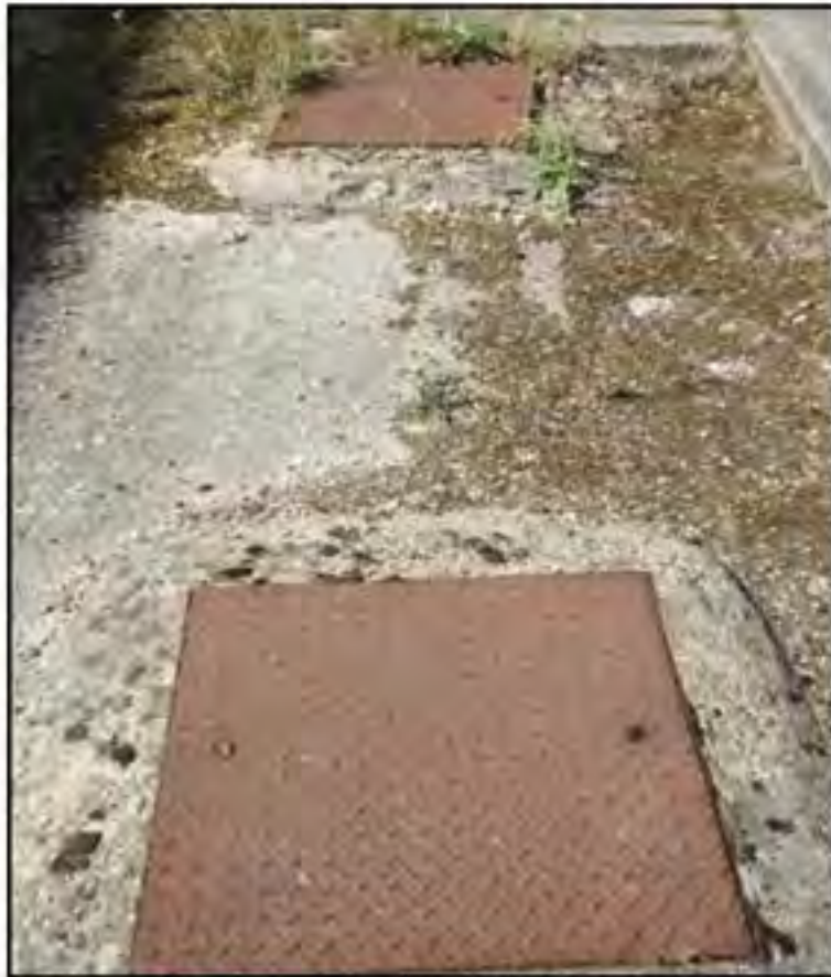
Plate 8: Manhole covers possibly indicating presence of interceptor or UST adjacent to Hangar 2.
