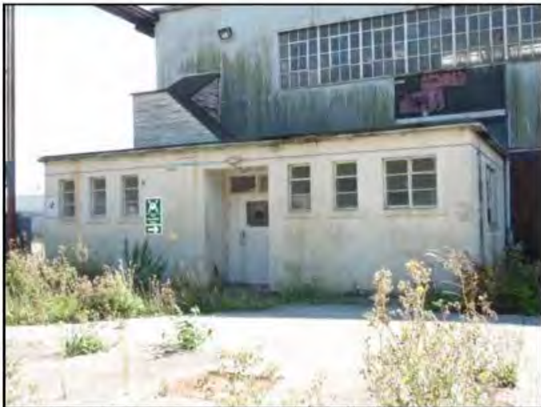
Plate 4: Building used as former oil stores on West side - Hangar 1.
