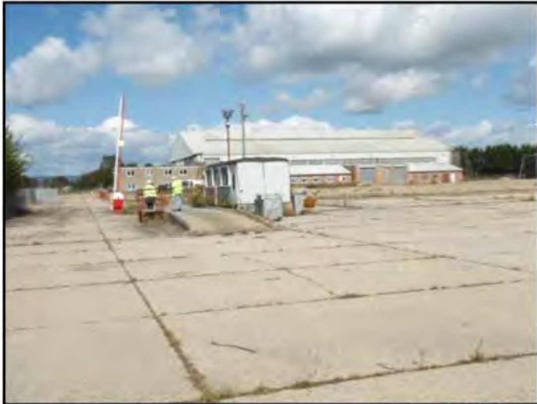
Plate 5: View of weighbridge looking North towards Hangar 1 - Aggregate Block Building.
