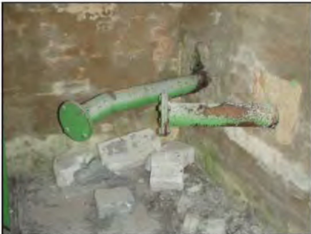
Plate 16: Redundant pipework inside the former RAF refuelling pumping station.
