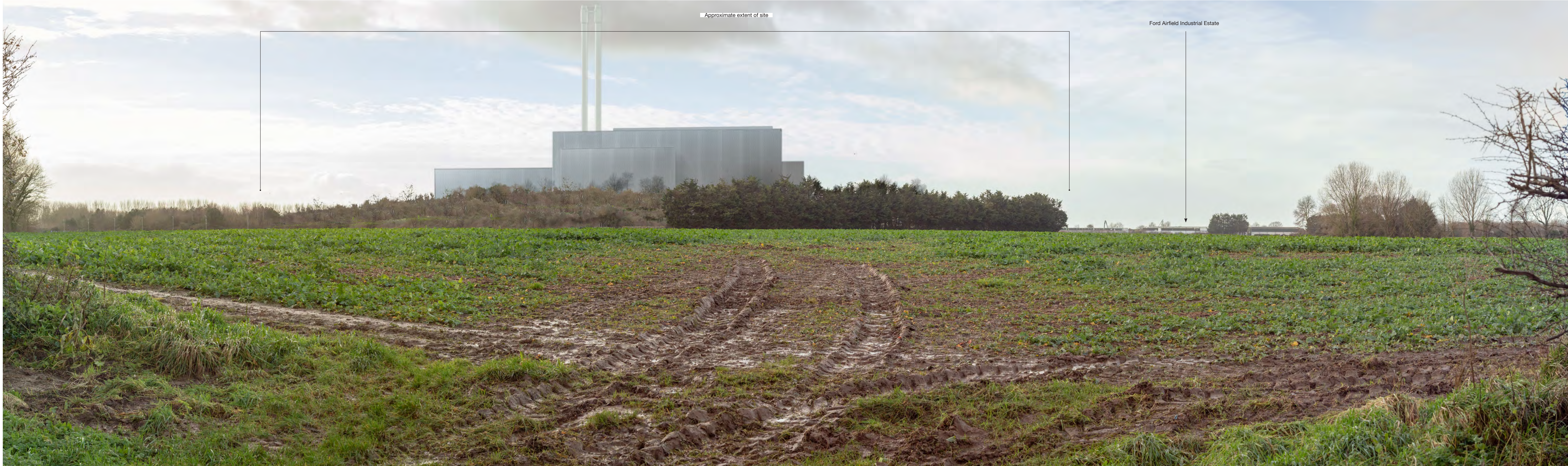
Viewpoint 26 from Ford Lane looking south toward site Visualisation type 4*. To be viewed at a comfortable arm's length and printed at A1 * Refer to Technical Appendix H for visualisation details
