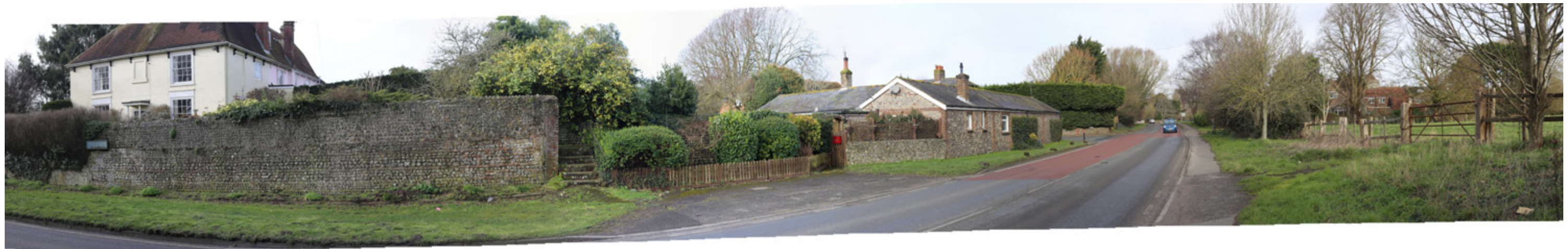
View of Church Farmhouse and along Ford Road including glimpses of the church tower
