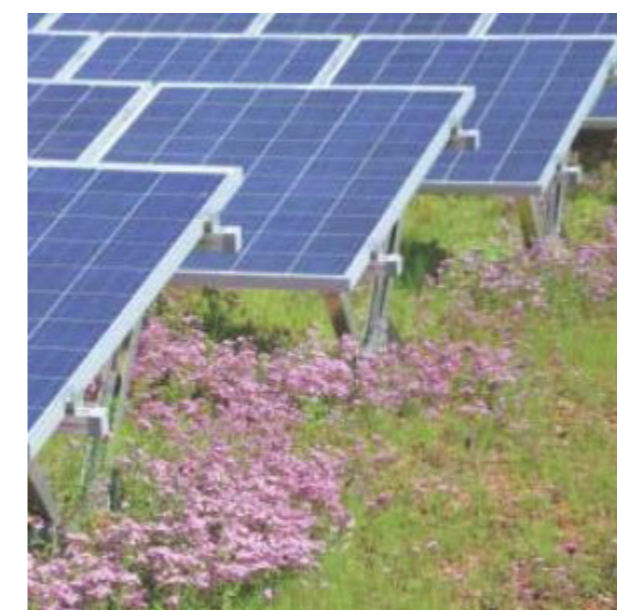
Bauder - Sedum blanket roof
