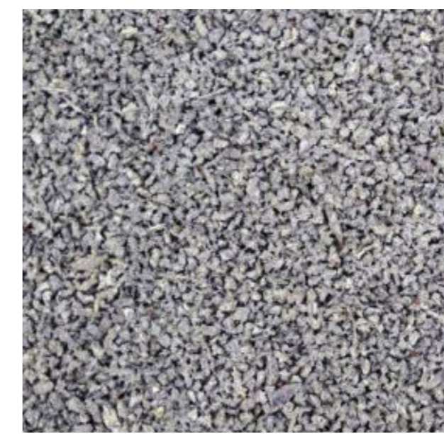
Wet pour/tiled rubber crumb to external terraces
