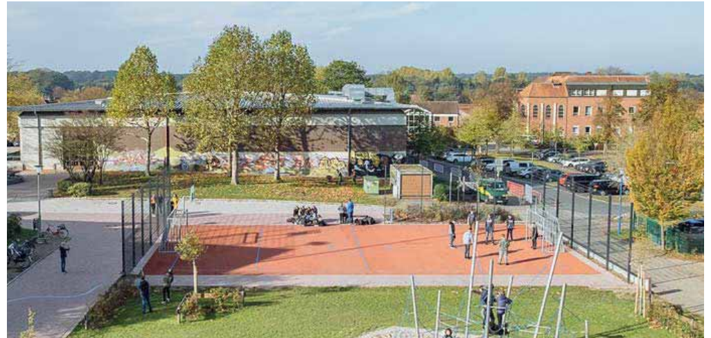
MUGA and adjacent playing field create a fun and high energy environment
