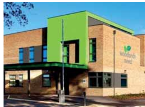
Existing School building
