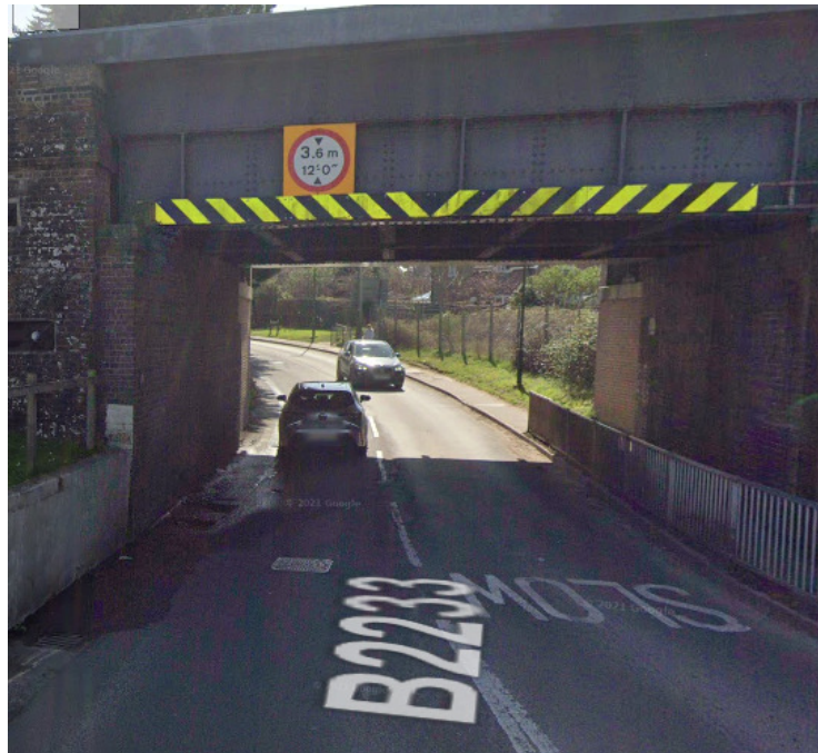
Figure 3 - Height Restriction Railway Overbridge on B2233 Barnham Road
