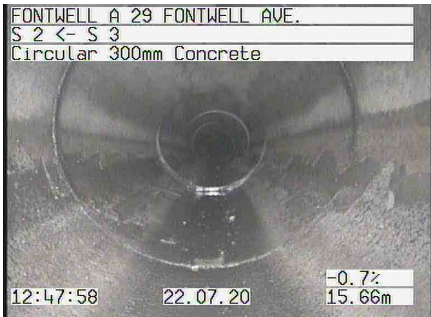
S 2X_63a01a65-f631-48db-947e-15d36b19dba8_20200722_124950_044.jpg, 00:02:04, 15.66 m
