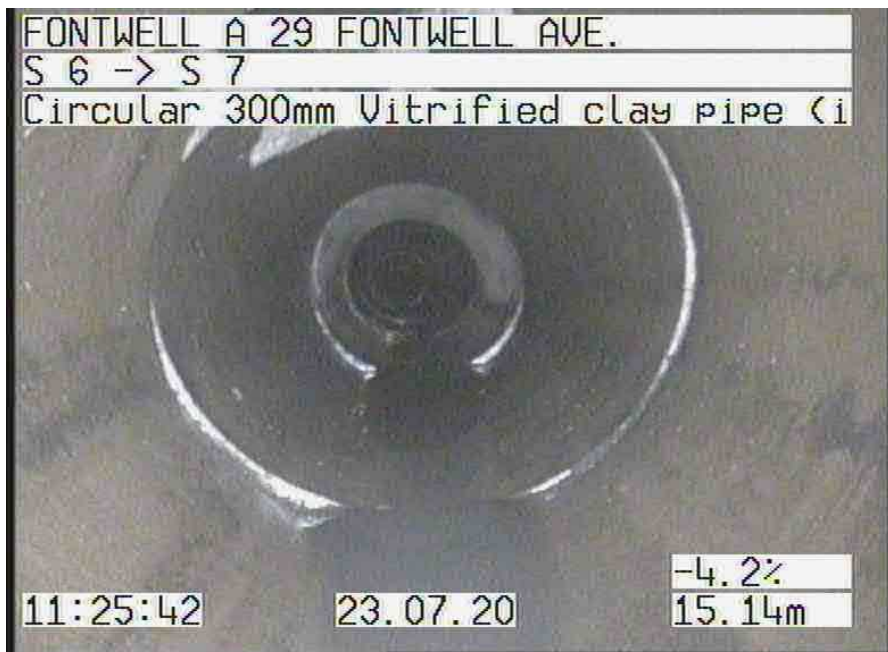
S 6X_20e5e42f-d214-462d-ae3a-a7277b04ff96_20200723_112721_561.jpg, 00:01:59, 15.14 m
