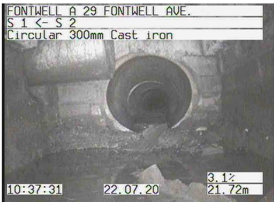
S 1X_e2bbe1f4-2f57-4af3-9f5a-b69f842627ae_20200722_103922_750.jpg, 00:01:48, 21.72 m Finish node type, catchpit, reference number: S 1
