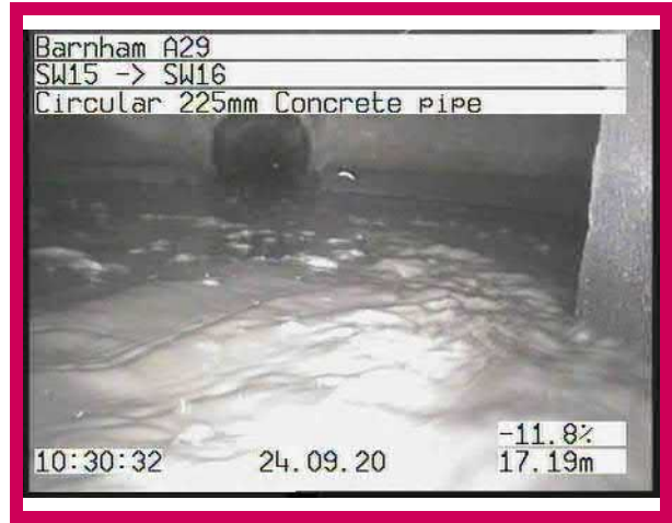
2, 00:01:40, 17.19 m Finish node type, catchpit, reference number: SW16
