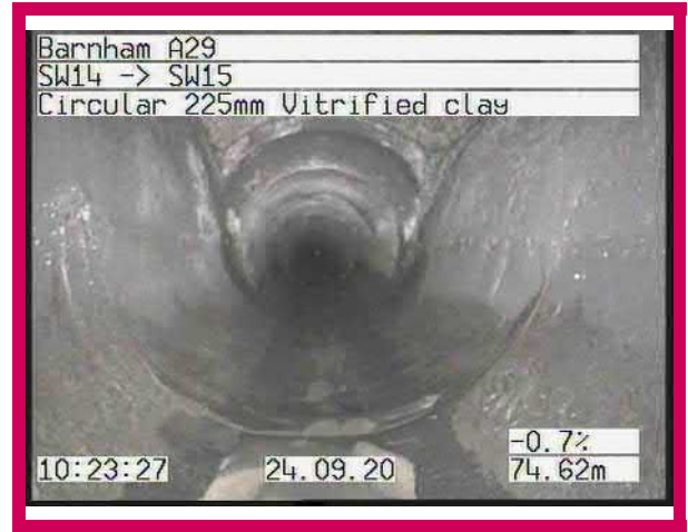
2, 00:06:09, 74.62 m Finish node type, manhole, reference number: SW15
