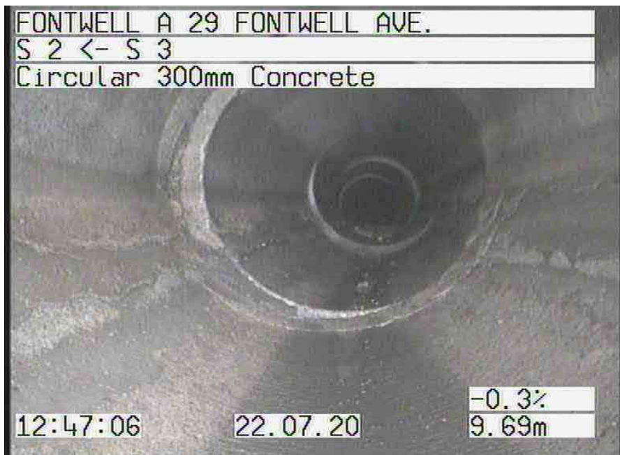
S 2X_05743cde-0a51-4426-b771-72a0ad369a01_20200722_124857_702.jpg, 00:01:27, 9.69 m
