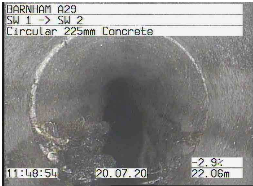
SW 1X_9a1ee07d-49b8-4700-bff9-324346e06c99_20200720_115041_009.jpg, 00:01:47, 22.06 m
