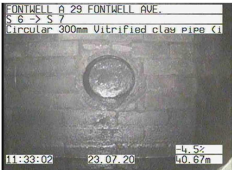
S 6X_d43505a4-c358-430b-9d72-d3a2464fef57_20200723_113441_080.jpg, 00:07:32, 40.66 m Finish node type, catchpit, reference number: S 7
