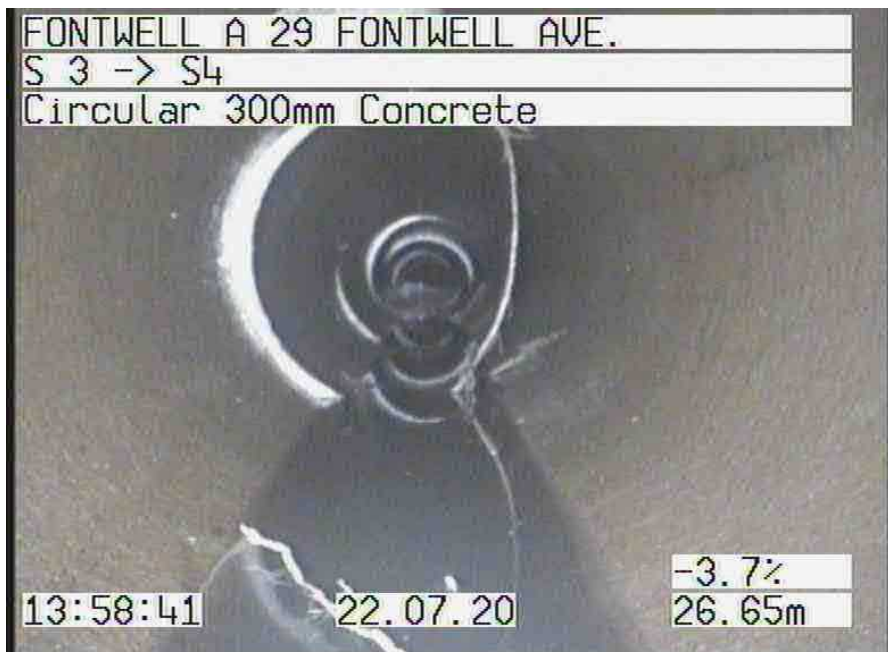
S 3X_c9aaf483-d7fb-402c-9b98-ad468d006810_20200722_140017_628.jpg, 00:03:25, 26.65 m
