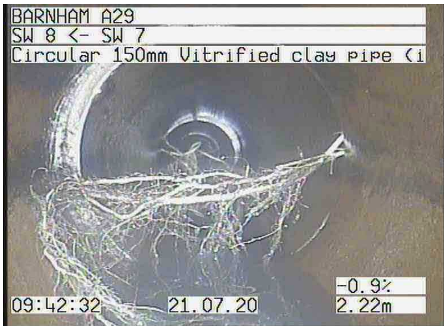
SW 8X_1b3da3de-c7a2-4ca9-87bb-f46f9c065640_20200721_094421_060.jpg, 00:00:39, 2.09 m Roots, tap at joint
