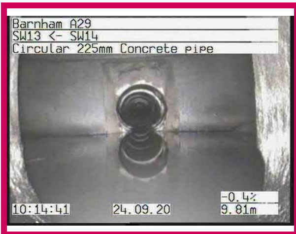
3, 00:01:14, 9.81 m Finish node type, catchpit, reference number: SW13
