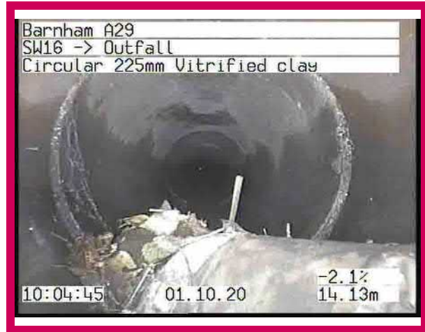
2, 00:01:36, 13.73 m Other obstacles from 4 o'clock to 8 o'clock, 25% cross-sectional area loss, debris
