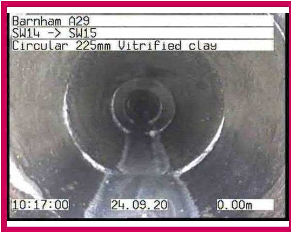
1, 00:00:11, 0.00 m Start node type, manhole, reference number: SW14
