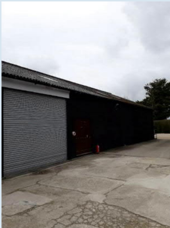
Photo 7. Northern aspect of building B7.
