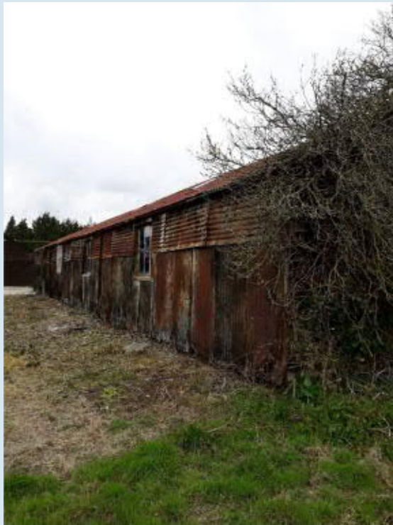
Photo 5. Southern aspect of building B5
