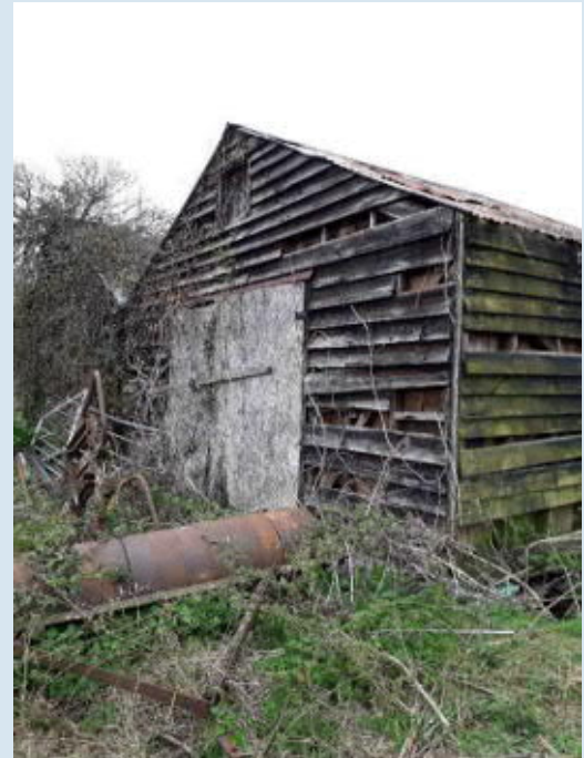
Photo 4. Eastern aspect of building B5
