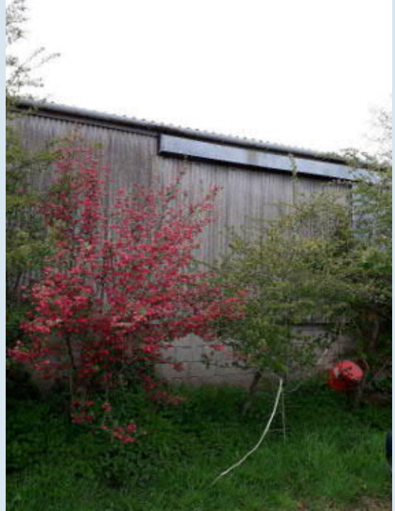
Photo 2. Eastern aspect of building B2
