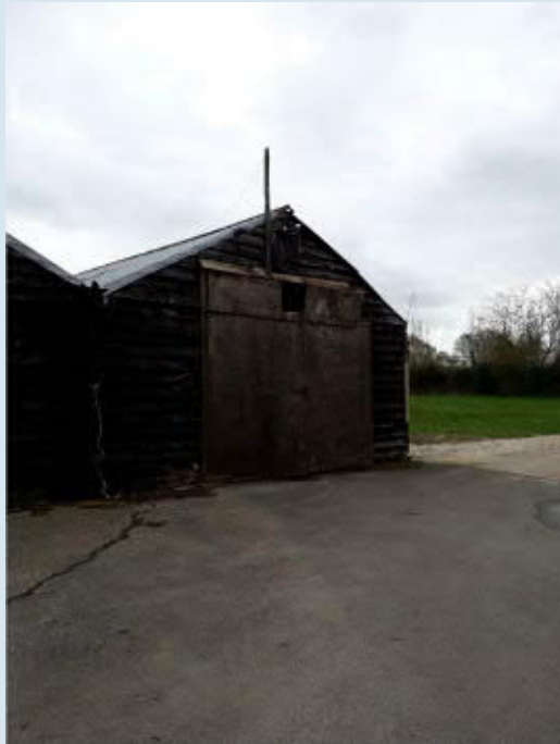
Photo 3. Western aspect of building B5
