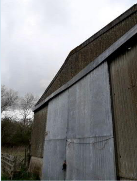
Photo 1. Southern aspect of building B2
