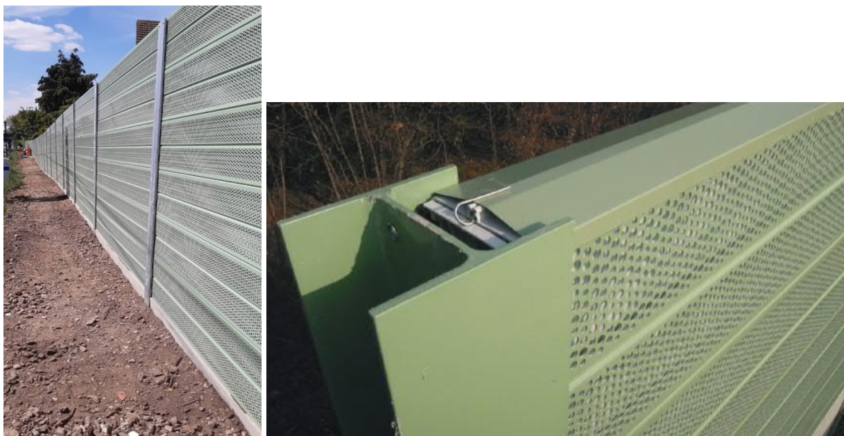
Figure 4-12 – Acoustic fence plastic ‘eco’ material
