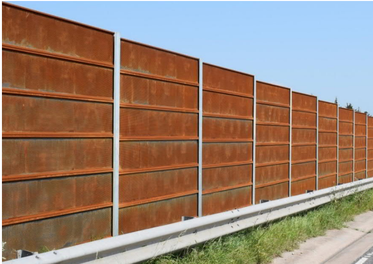
Figure 4-10 – Acoustic fence weathering steel finish
