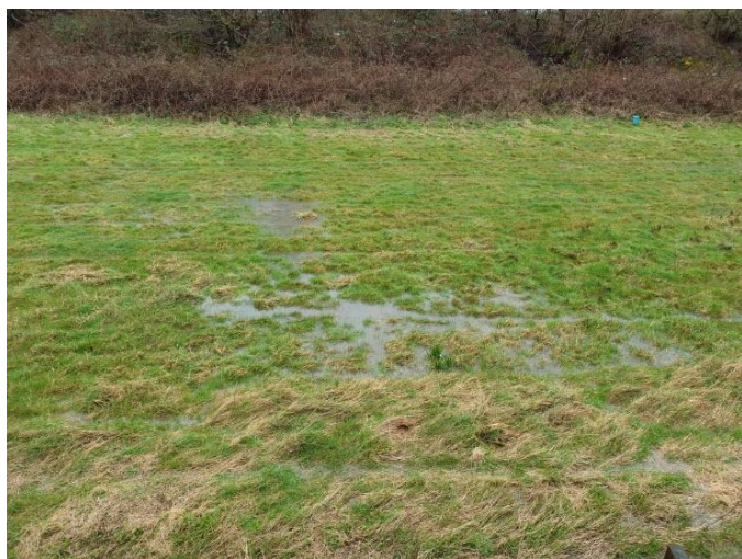
3 rd March 2020 – most recent flooding
