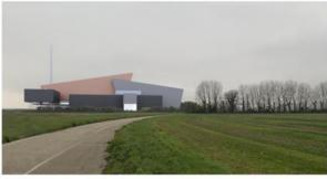
The facility would see 275,000 tonnes of non-recyclable waste per year burned at high temperatures to generate 28MW (net) of energy.
