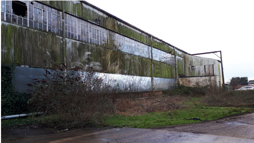
Photo 3. Hangar 1, facing southwards
