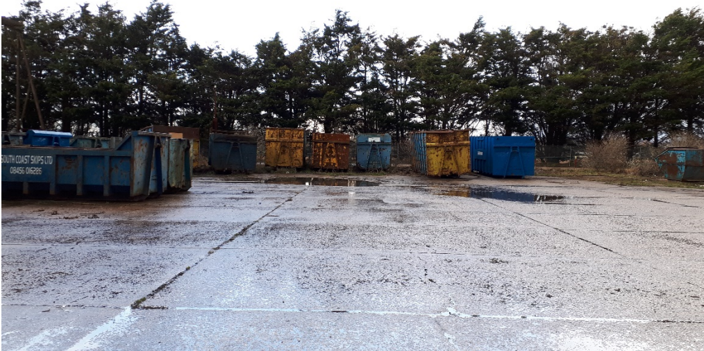
Photo 7. Yard area, facing northwards
