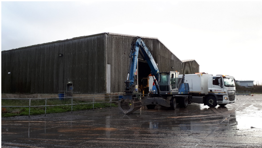
Photo 6. Main waste building
