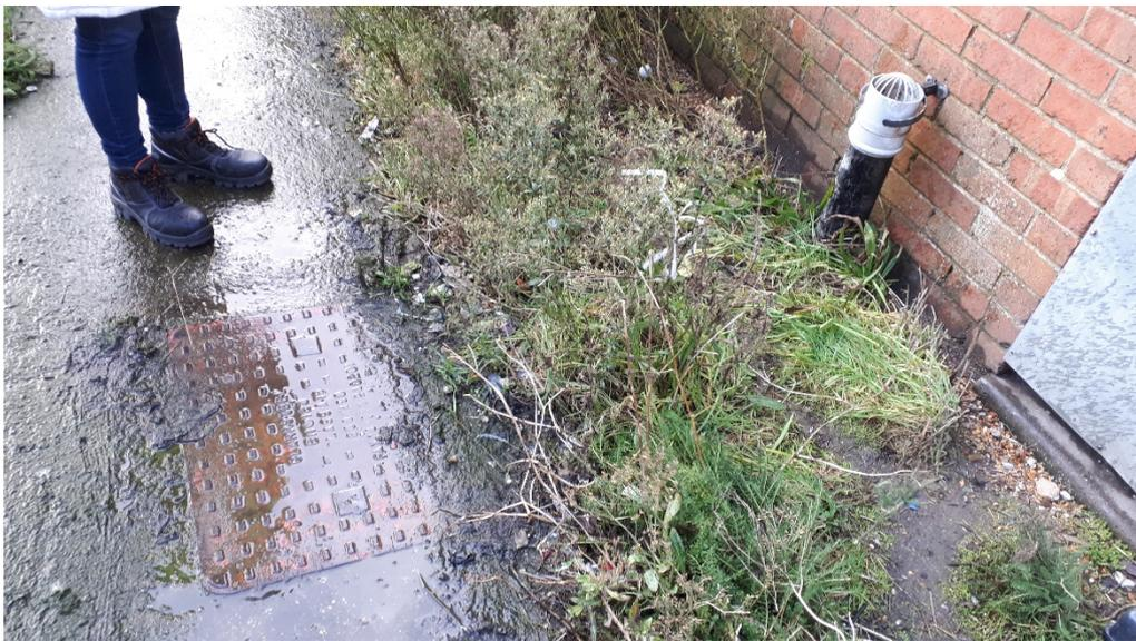
**Photo 14.** Cover Possibly Indicating the Presence of an Interceptor or Underground Storage Tank Adjacent to Hangar 2
