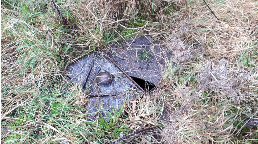
**Photo 13.** Cover Possibly Indicating the Presence of an Interceptor or Underground Storage Tank Adjacent to Hangar 2
