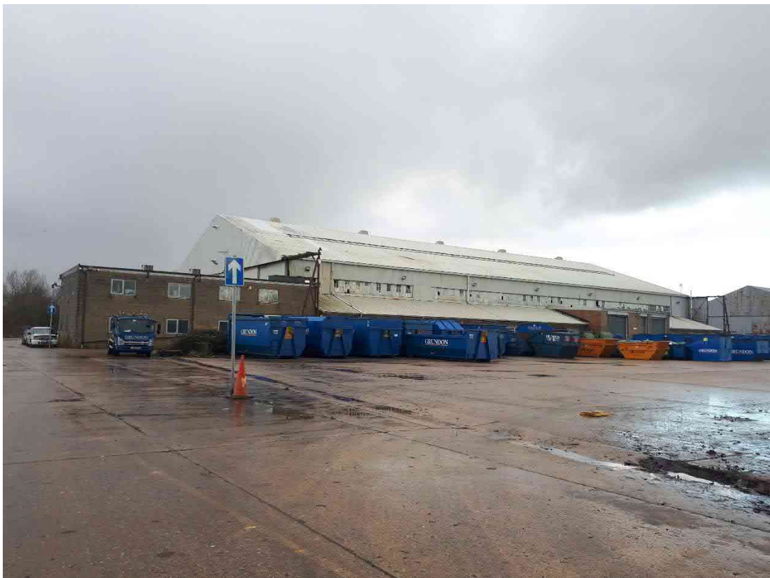
Photo A.2: View of Unit 1 (Hangar 1)
