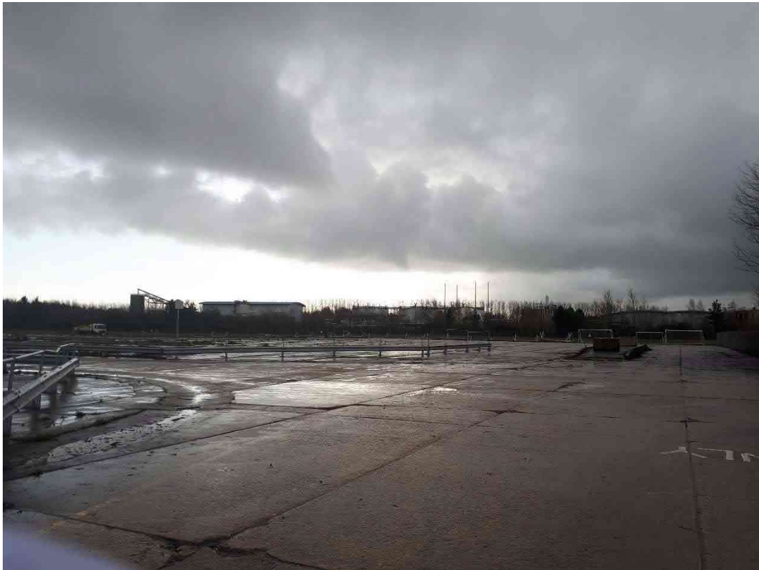
Photo A.1: View from the southeast corner of the site
