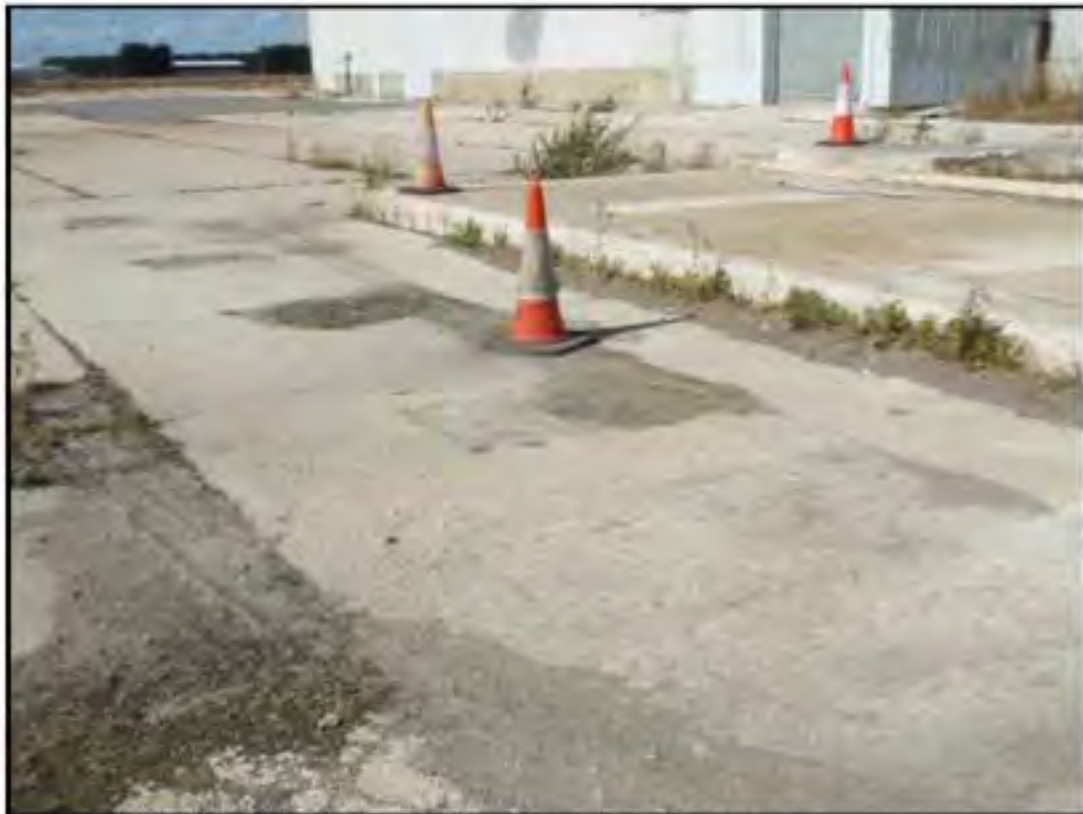
Plate 2: Location of Former boiler house gas oil tank (60,000 litres).
