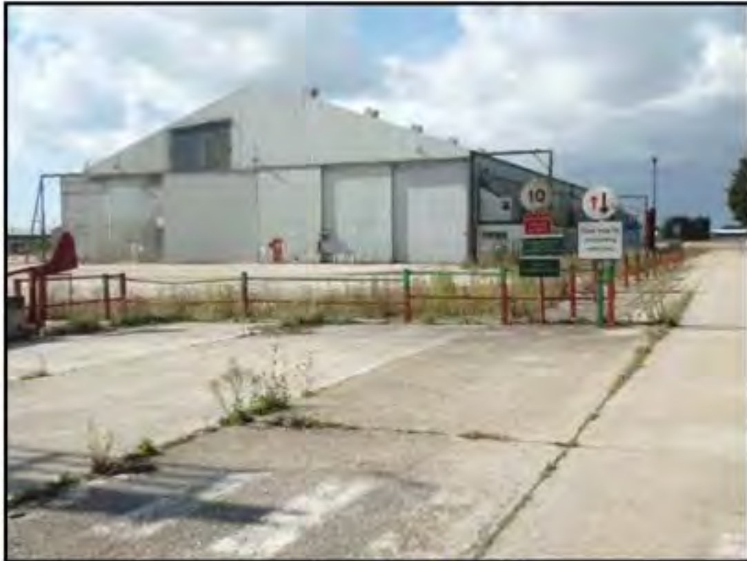
Plate 1: View looking West towards Hangar 1 along access road.
