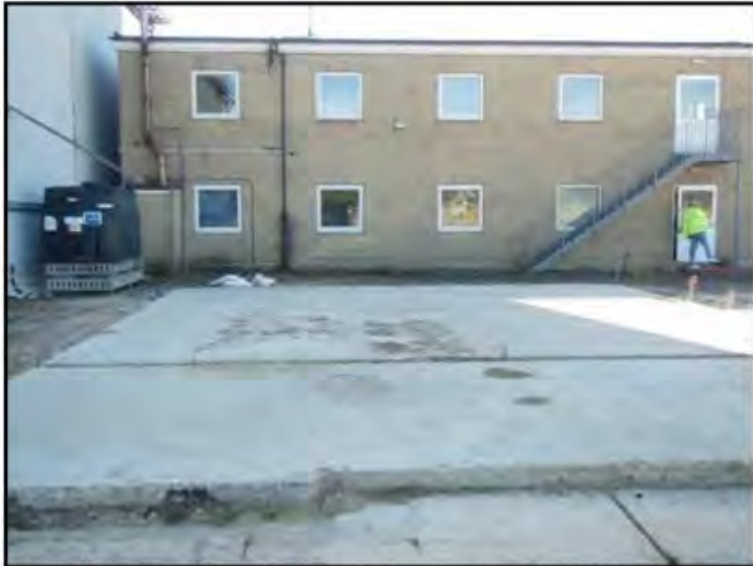
Plate 3: Above Ground Storage Tank previously containing gas oil (2,500 litres).
