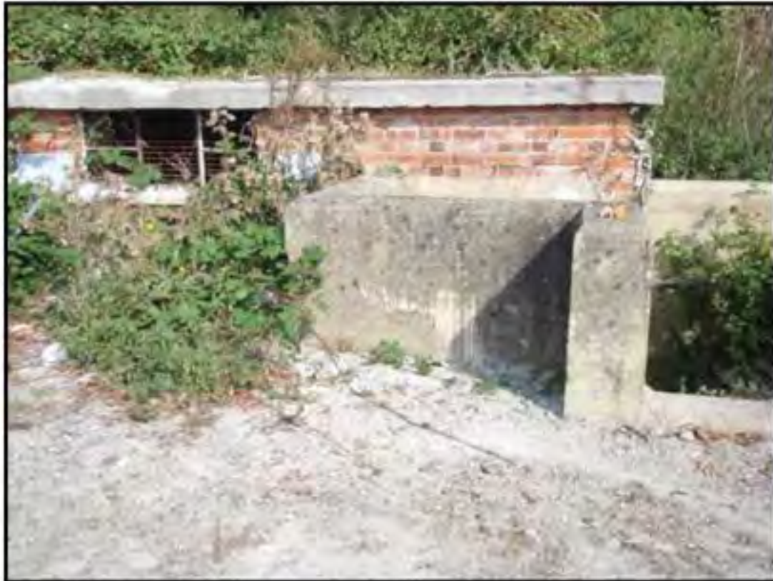
Plate 15: Former RAF refuelling pumping station.
