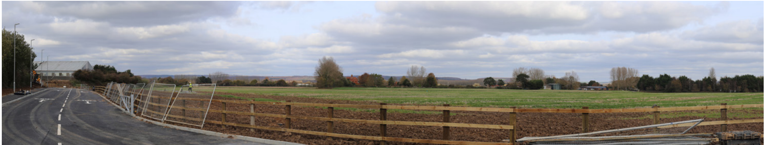
The new access road under construction, and view towards the rear of the buildings along Ford Lane
