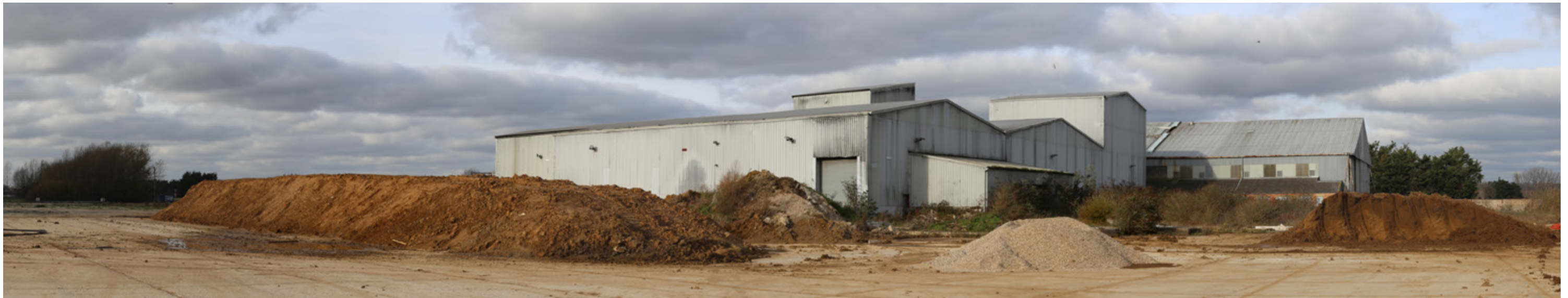
The B1 hangars and other buildings on the site
