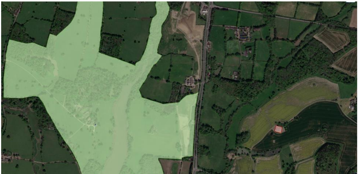
Image 19 Aerial view showing the Moated Site in West Grinstead Park (pink) in relation to the A24 and the Registered Knepp Park with the earthworks of the consented 2012 scheme visible. The moated site lies in a stand of trees south of Green Lane.
