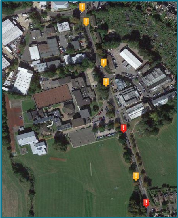
Figure 3.2 – Northerly Section of Imberhorne Lane
