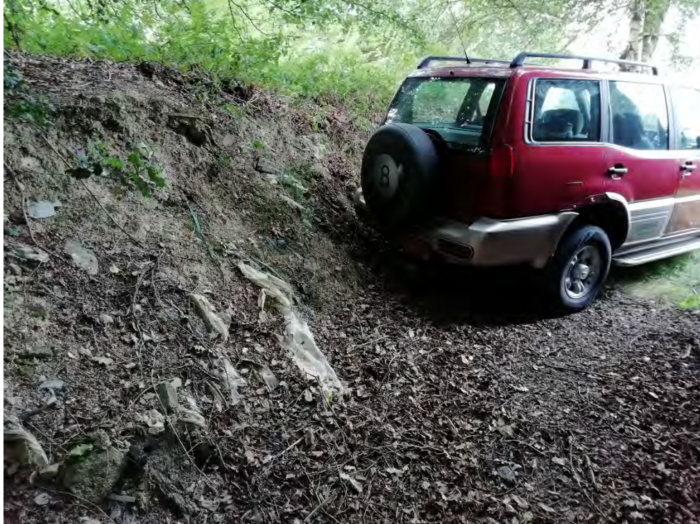
Plate 37 – Embankment next to wood store
