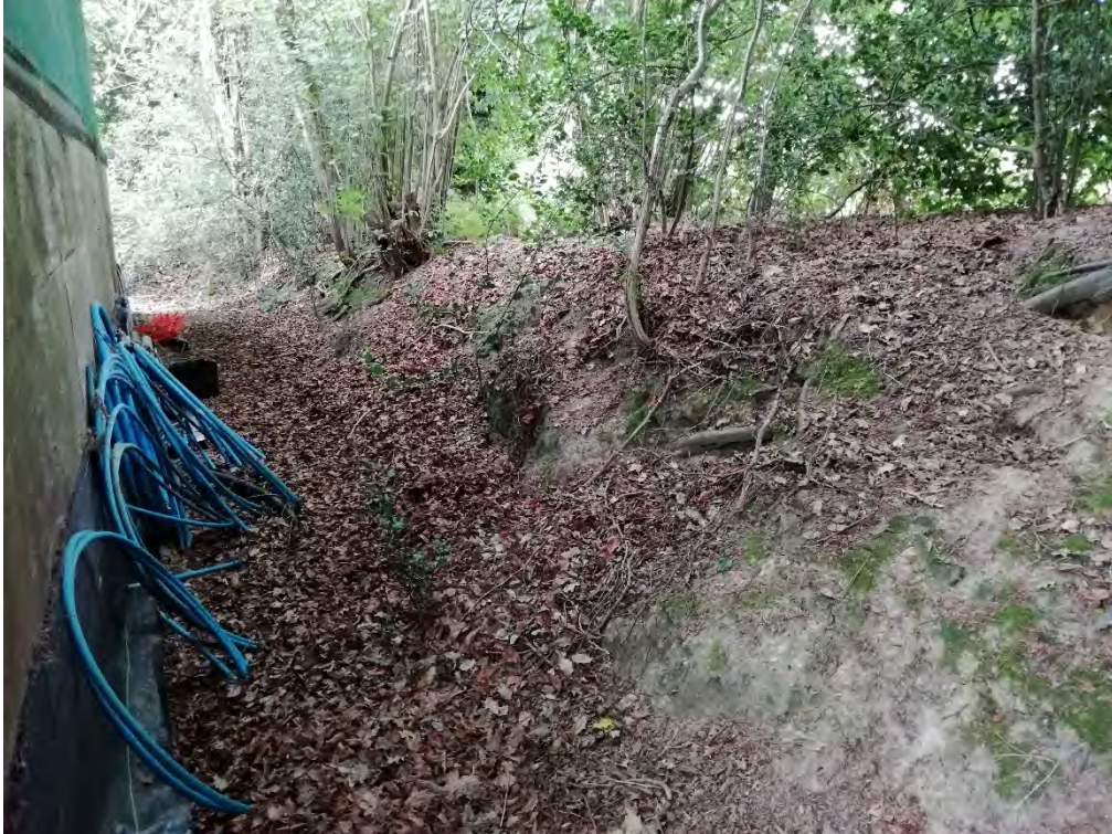
Plate 35 – Embankment behind wood Store
