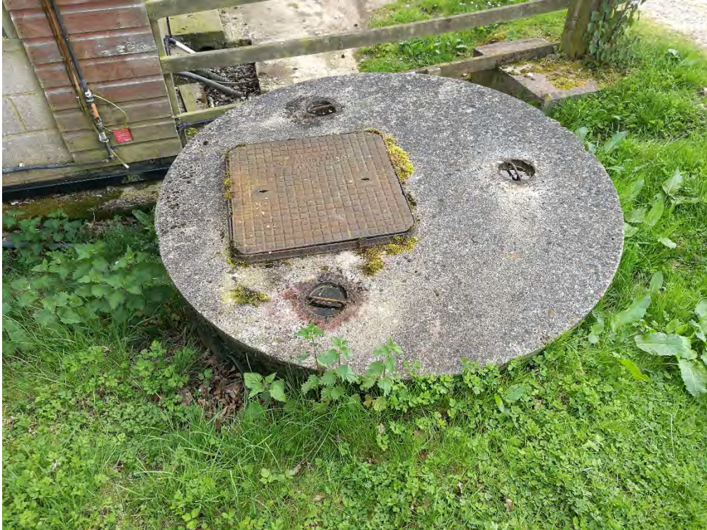
Plate 33 – Services on site
