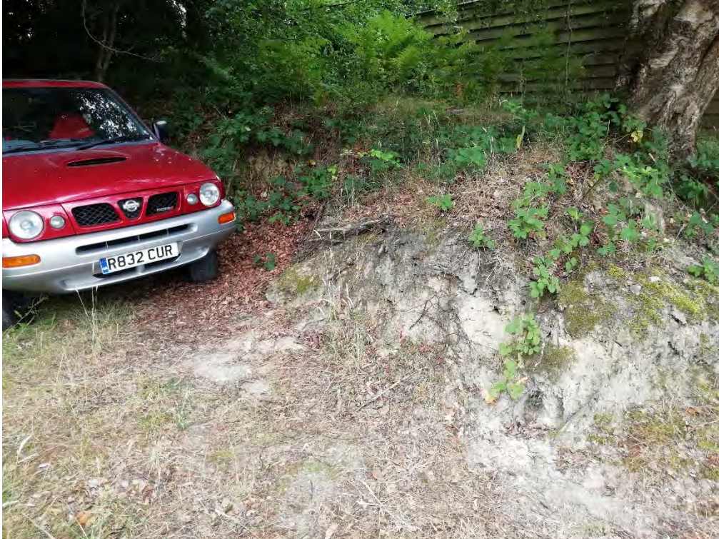
Plate 39– Embankment next to wood store
