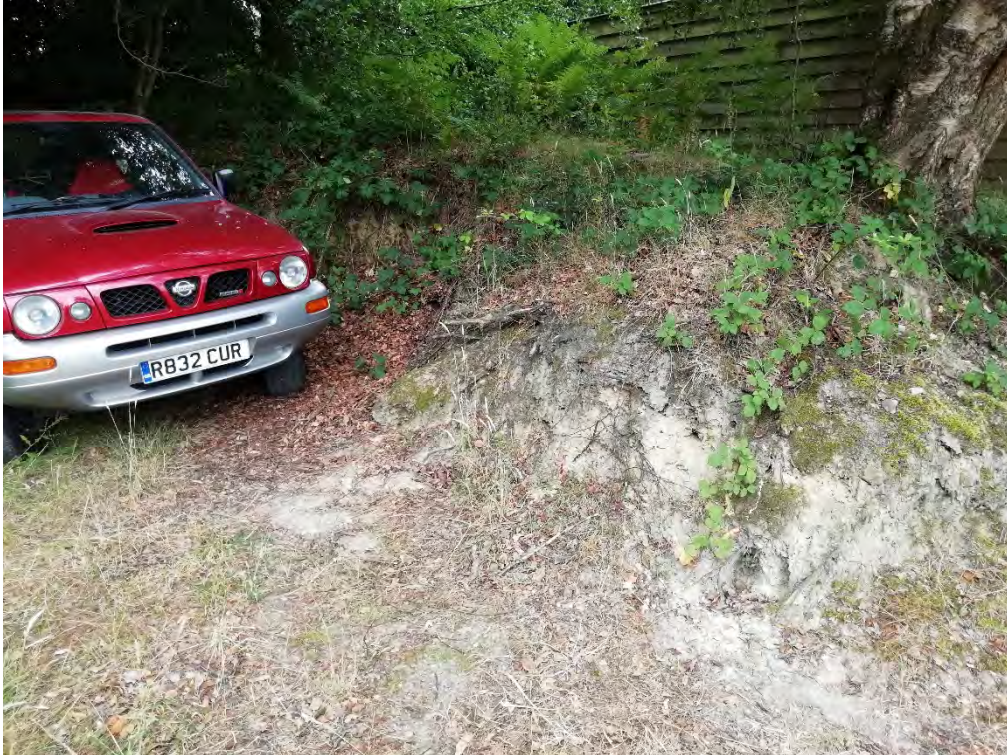
Plate 39– Embankment next to wood store
