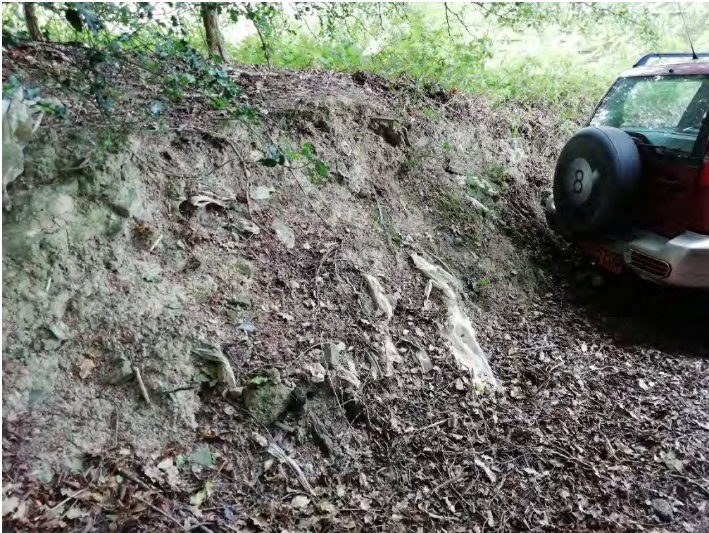
Plate 36 – Embankment next to wood store
