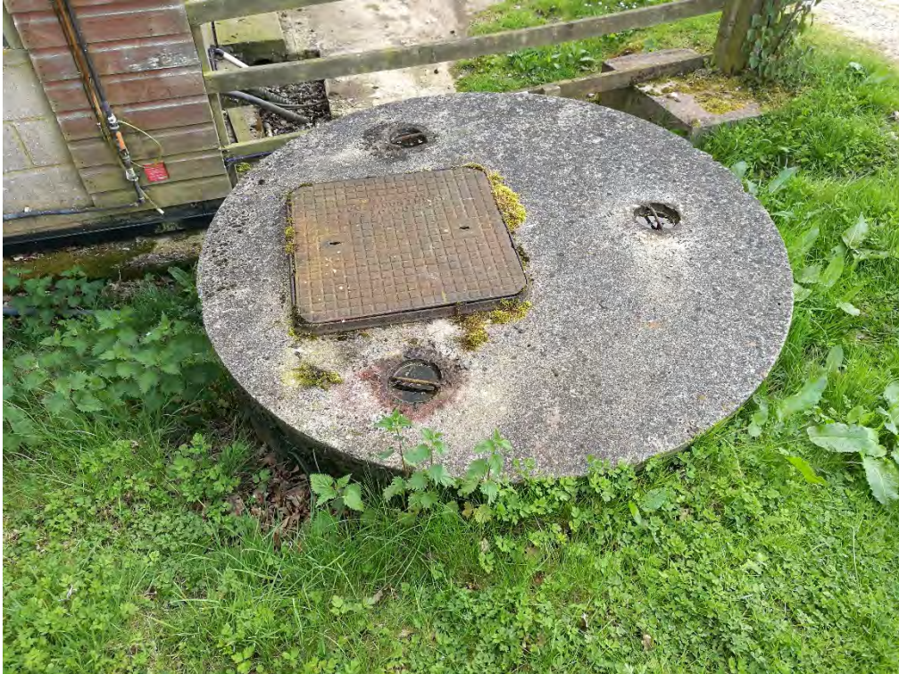
Plate 33 – Services on site
