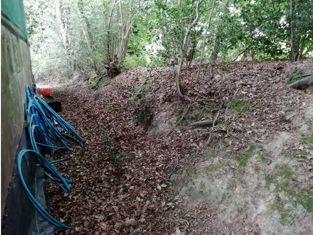
Plate 35 – Embankment behind wood Store
