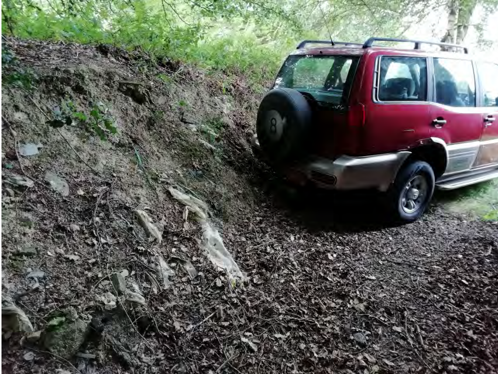
Plate 37 – Embankment next to wood store
