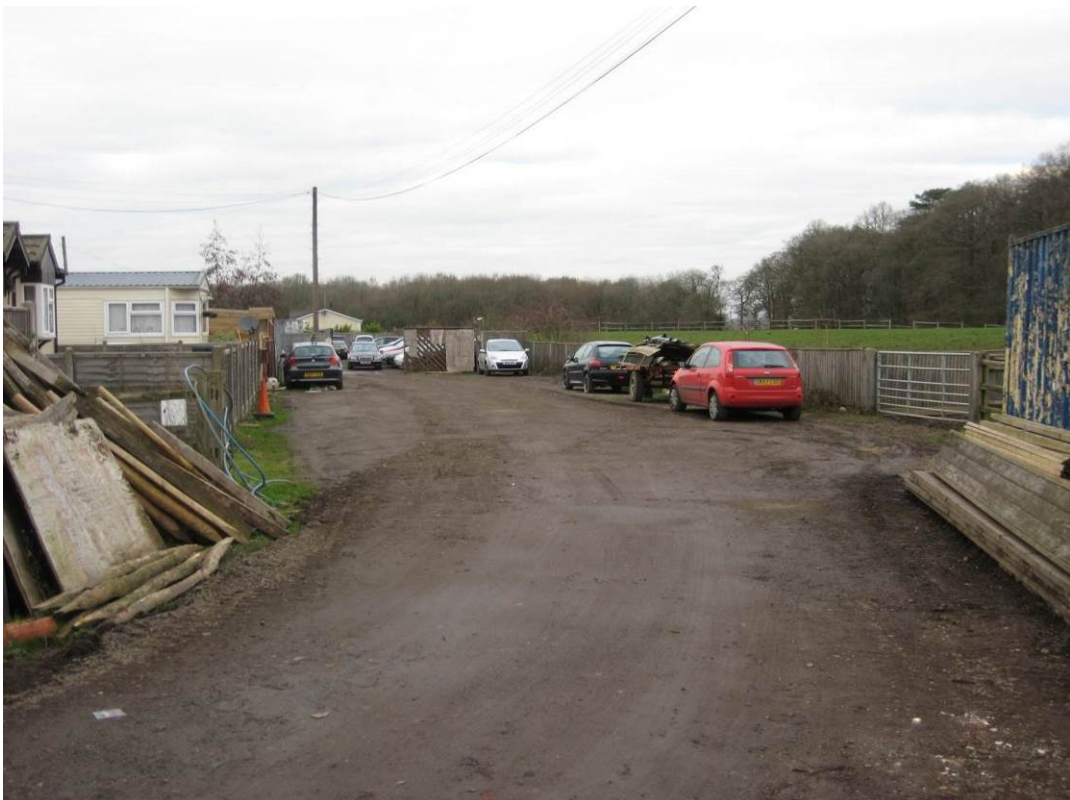
Photograph 2: Existing Site eastern side and the location of proposed a Soil Recycling and Concrete Crushing Facility
