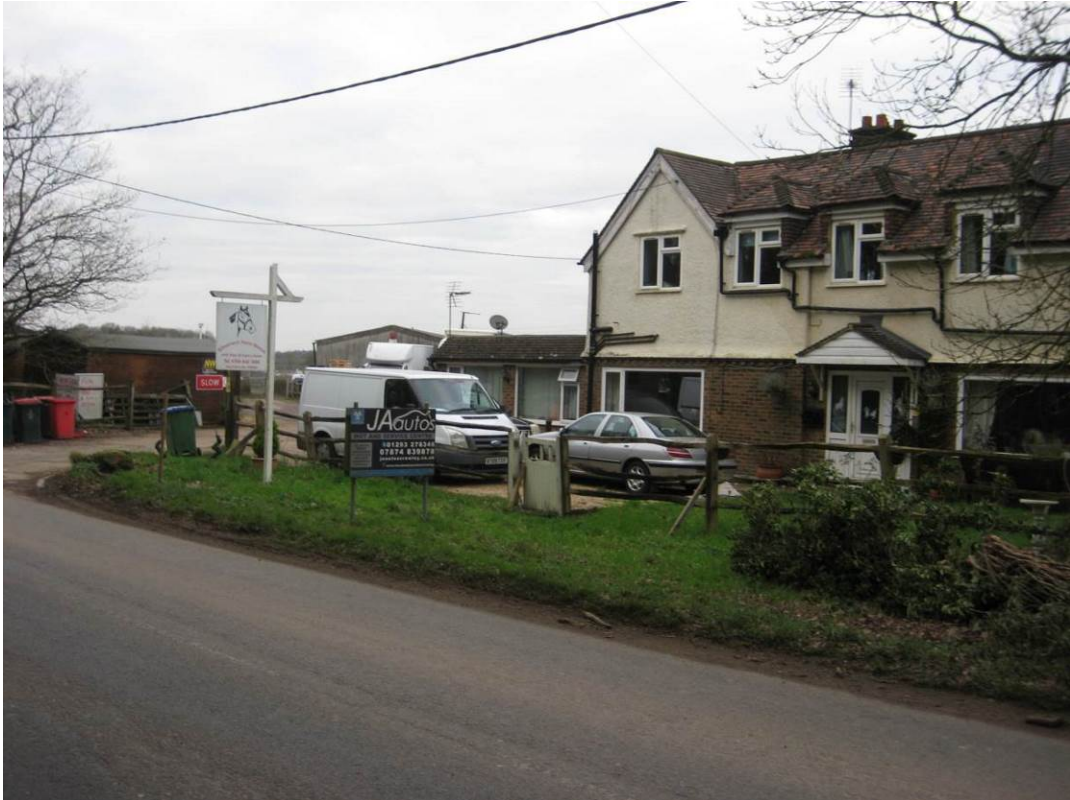
Photograph 1: Existing Site frontage viewed from Charlwood Road showing existing dwelling, stabling and storage areas
