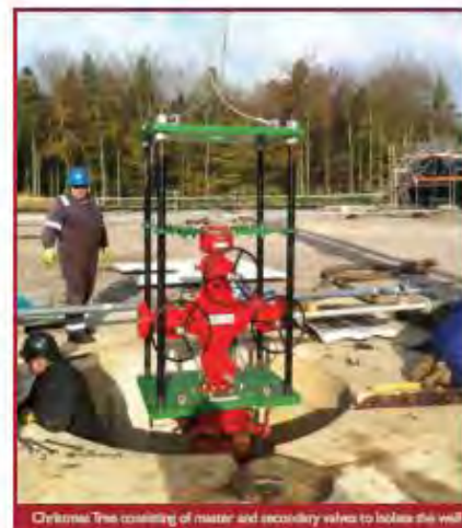
Onshore The casing of master and secondary valves to isolate the well
