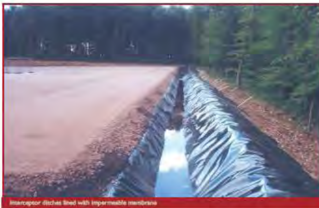
Interceptor ditches lined with impermeable membrane
