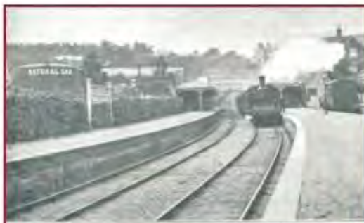
Discovery of Natural Gas in Sitons—Heathfield Station
