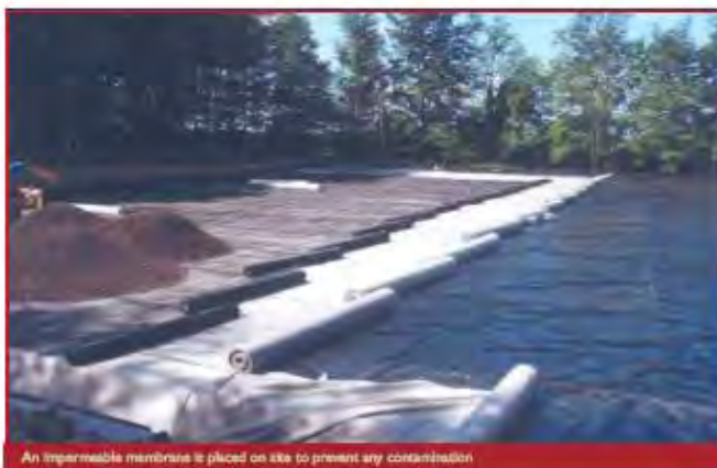
An impermeable membrane is placed on site to prevent any contamination
