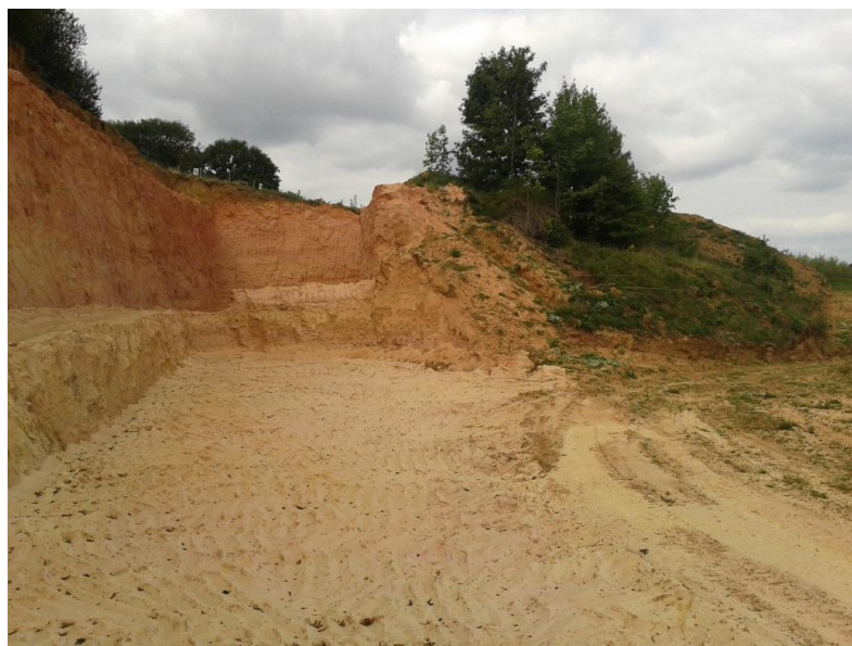
Figure 2 Western Extent of Excavation
