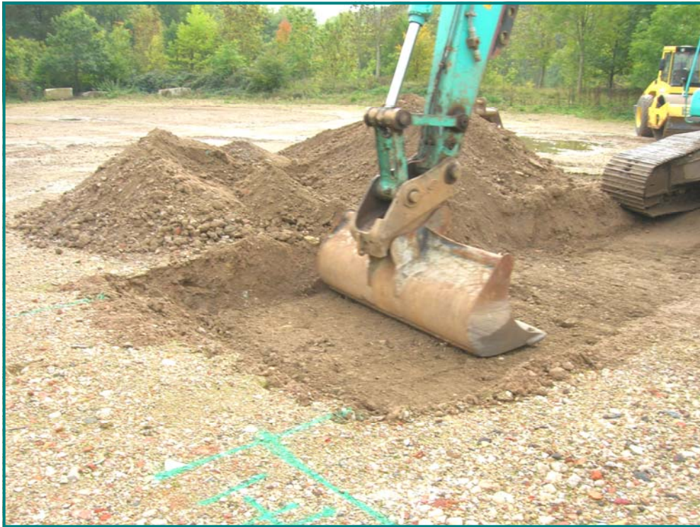
Photograph Location 7 — Trial fill trench 4th October 2010
