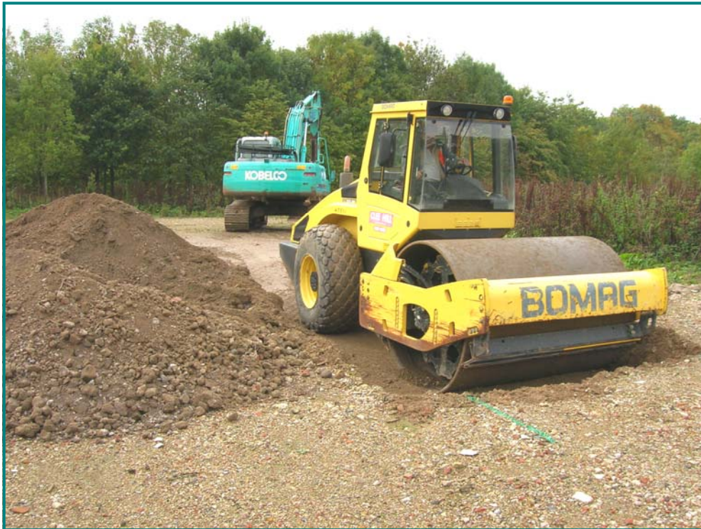
Photograph Location 13 — Trial fill trench 4th October 2010
