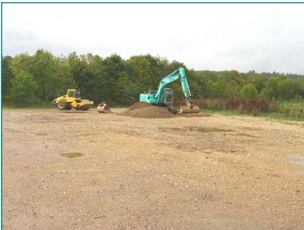
Photograph Location 14 — Trial fill trench 4th October 2010
