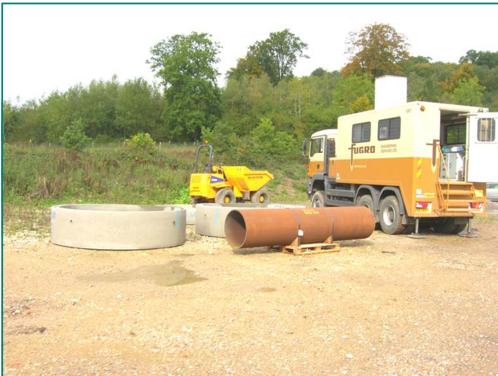
Photograph Location 6 — CPT test location 9 4th October 2010
