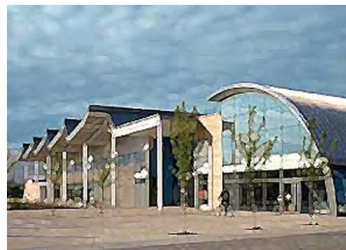
This award winning development highlights how different roof forms and materials within the same building can signify and welcome different types of user. The angular accented roof shapes supported by large pillars are functional and obvious as an industrial space accommodating vehicles, whilst the curved roof section, with its glazed facade has a pedestrian scale entrance. It also shows how a single building can successfully segregate a delivery area thereby minimising conflict
