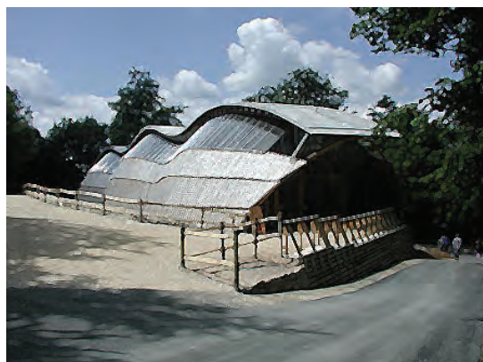
The Downland Gridshell highlights how the use of innovative designs can accommodate buildings which require a large roof form within a rural setting.
