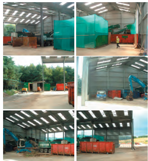
Heavy plant and large throughput mean sufficient space and height is necessary within enclosed waste transfer stations.
