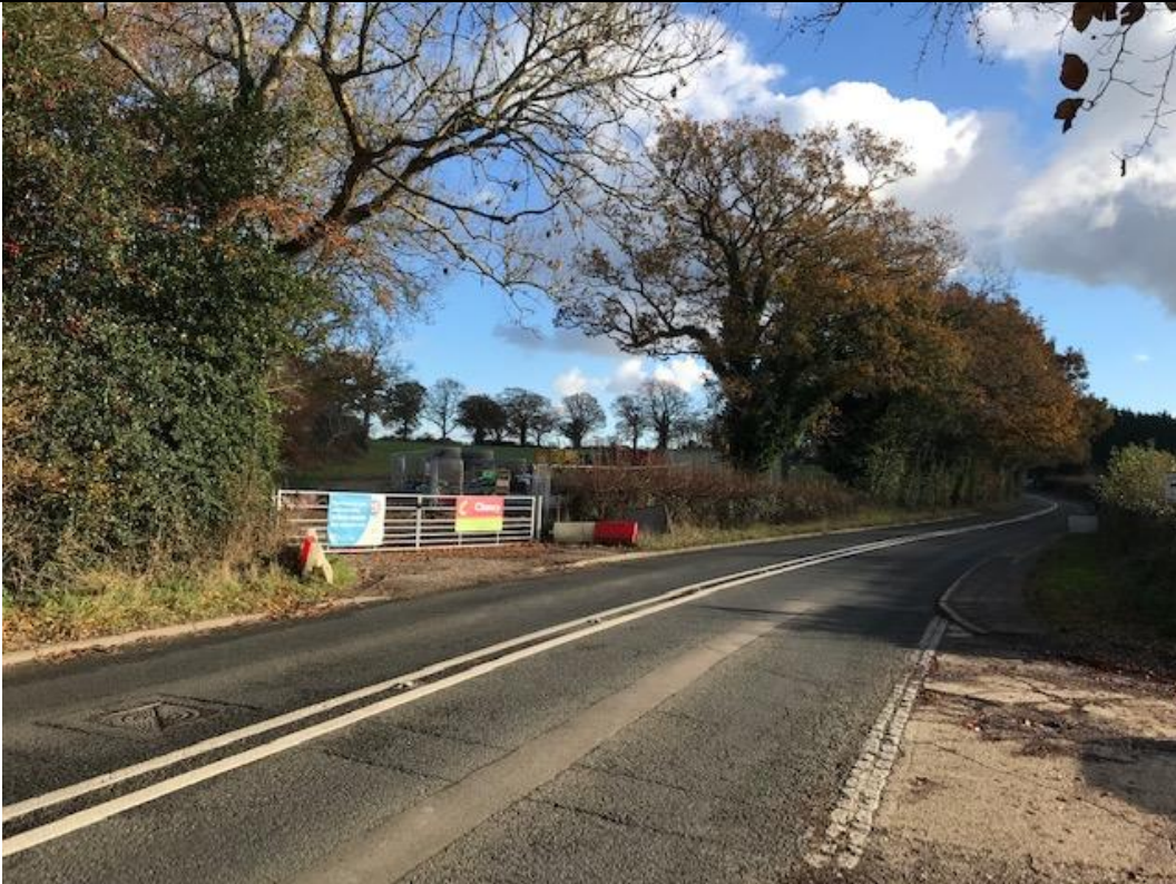
Image 1: Widened access as of 28 th November 2023
