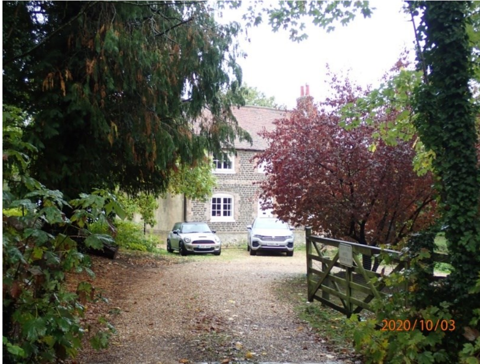
Plate 4: View of the Grade II listed Sandhill Farmhouse, (Site No. 22), from the south
