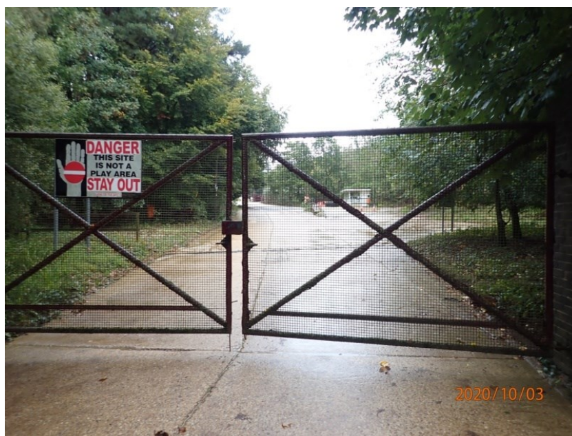
Plate 13: View of the entrance to Area B of the assessment sites, from the south-west
