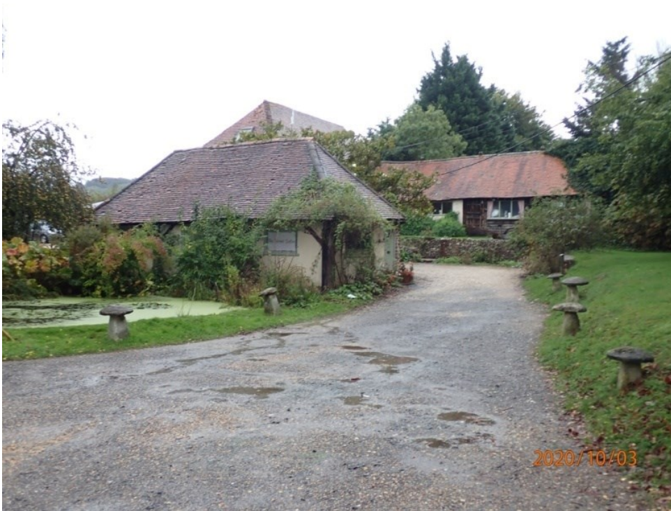
Plate 1: View of the outbuildings of the 18th century farmstead at Green Farm, (Site No. 47), from the south-west
