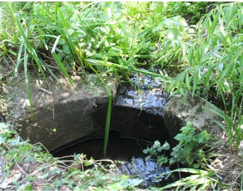
**Photograph B.** Curved brick wall structure, with flow focused to the centre holding the Honeybridge Stream, upstream of that culverted under the western end of The Pike, east of London Road.
