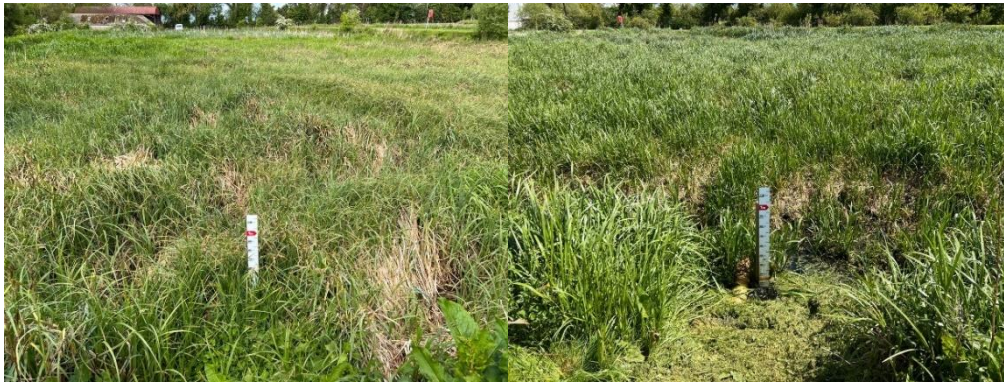
Figure 4: Before and after image of cleared vegetation around outlet pipe.
