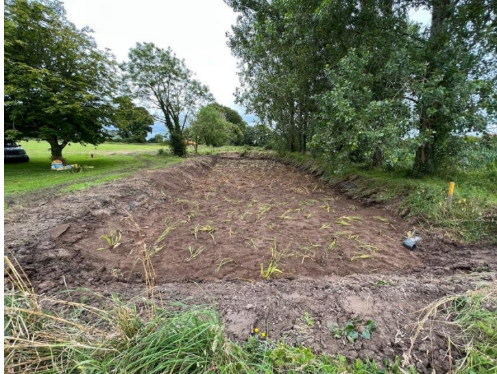
Figure 9: Wetland cell after de-sludging, addition of new topsoil and replanting.
