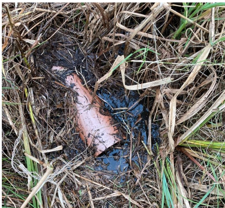
Figure 3: Example of blocked and overgrown pipe and cleared pipe.
