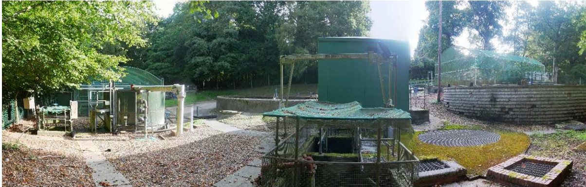
Photo 4 Mannings Heath WWTW
