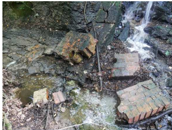
Photo 3 Headwall collapse
