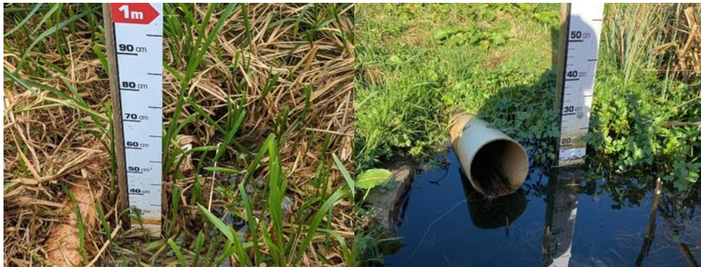
Figure 3: Examples of cleared vegetation from around outlet pipes.
