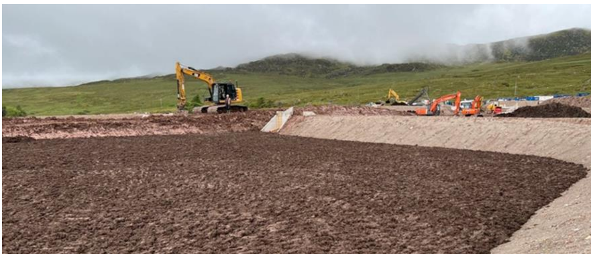
Figure 1: Topsoil over wetland cell base, ready for planting.
