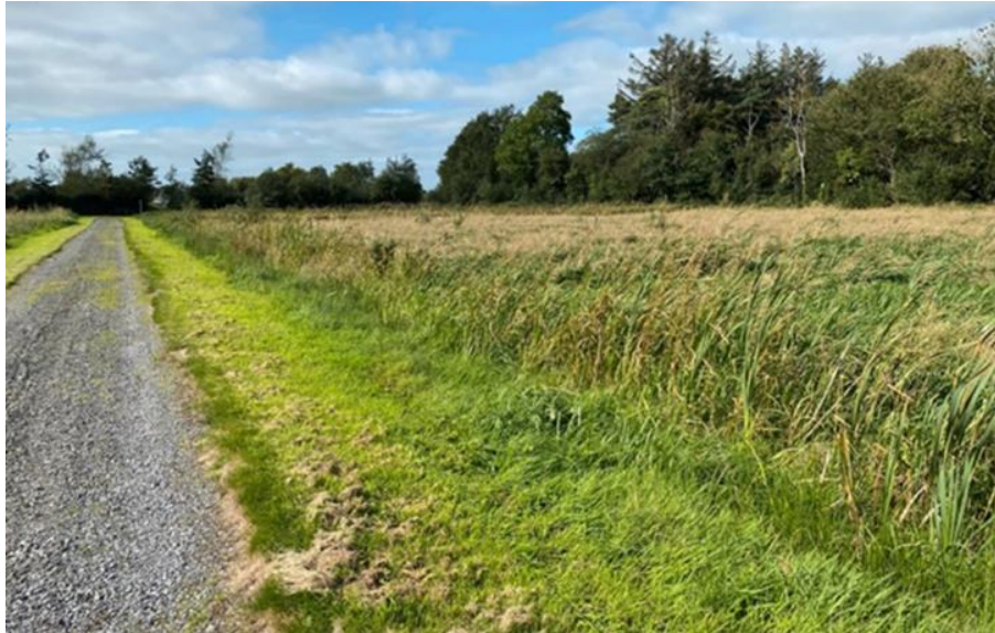
Figure 4: Mowed tops of embankments.
