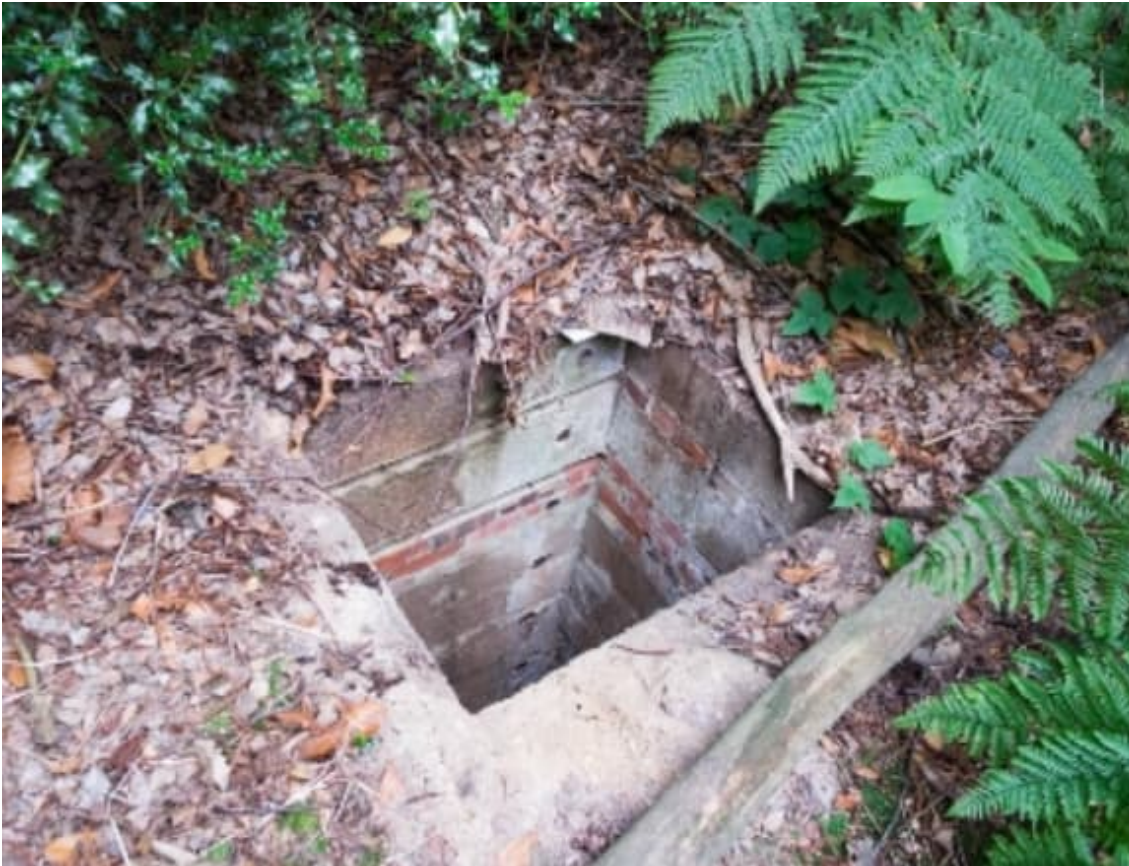
Photo B.4: Entrance to Staplefield Operational Base
