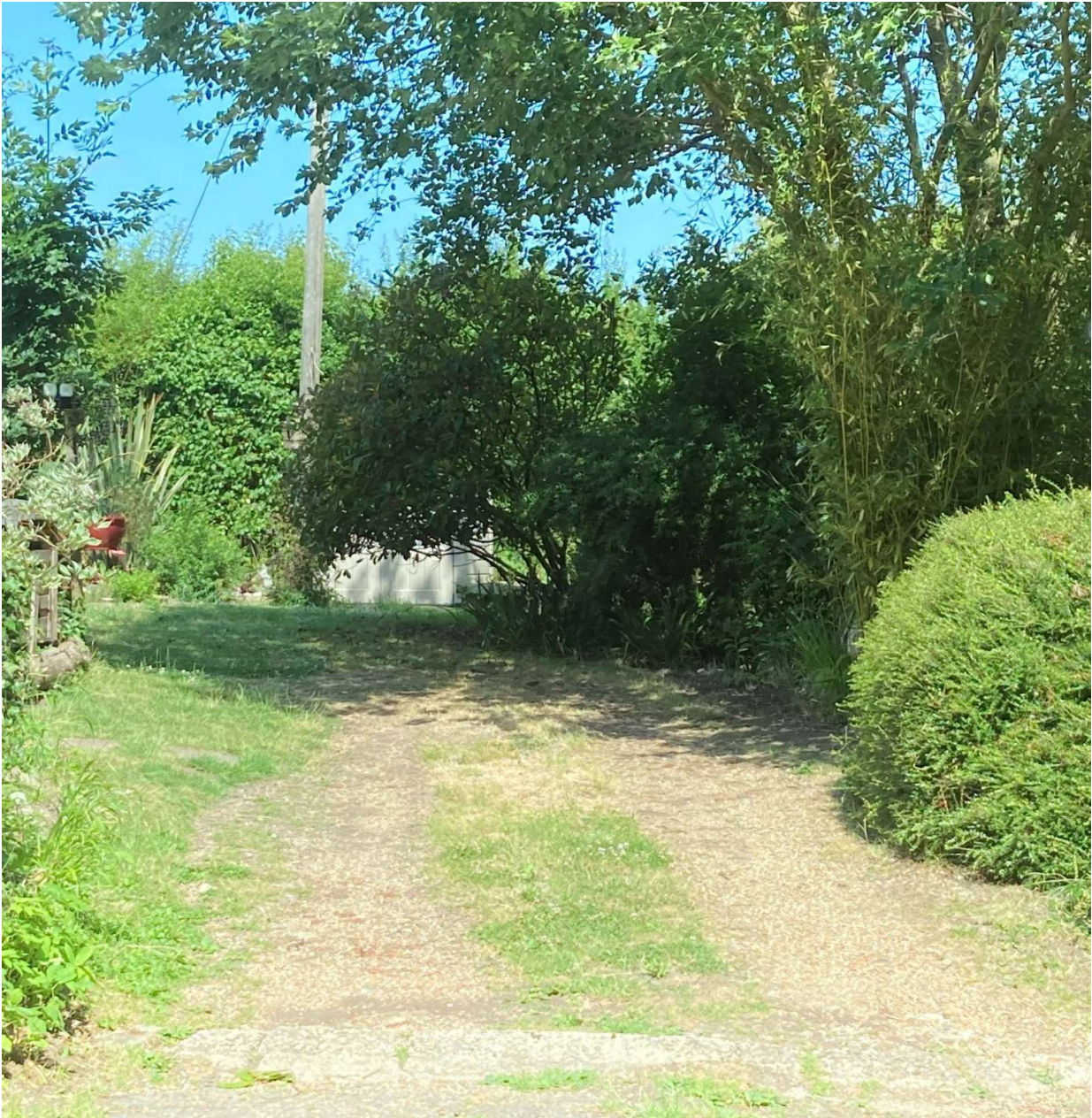
Plate 9 - Land to the east of No.2 Hooklands Lodge, where the vegetation will be removed to connect London Road to the temporary haul road.
