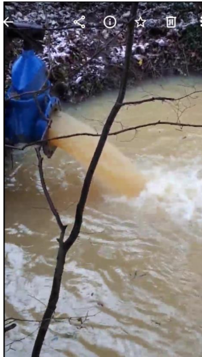
Silted water discharged to stream (January 2021)
