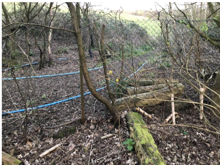
Leachate being processed and pumped back into the landfill site without monitoring or telemetry
