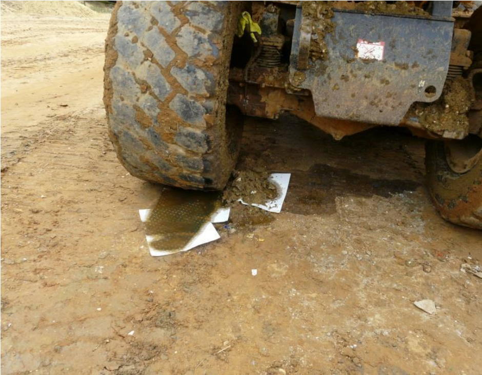
Leaked hydraulic fluid (May 2015)
