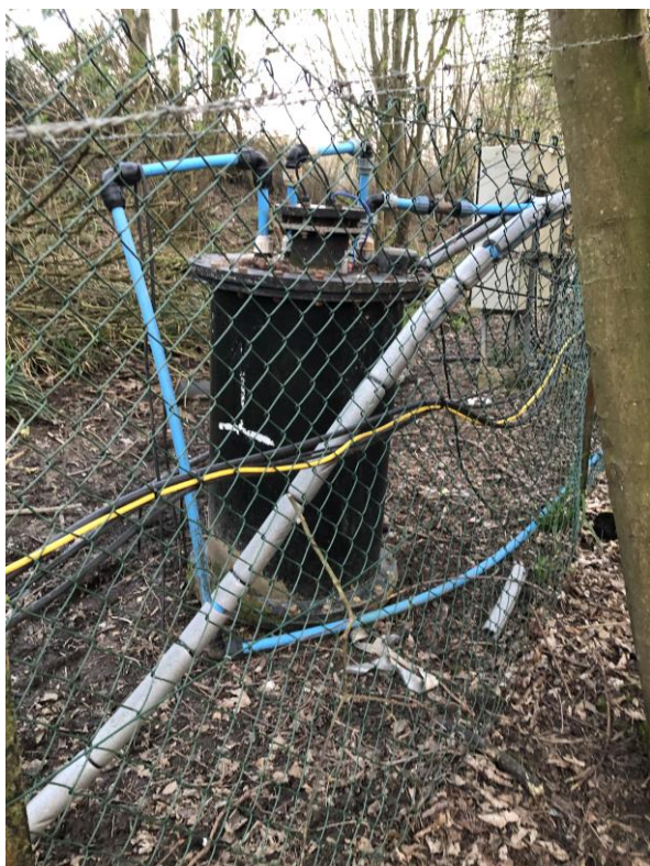
Leachate being processed and pumped back into the landfill site without monitoring or telemetry
